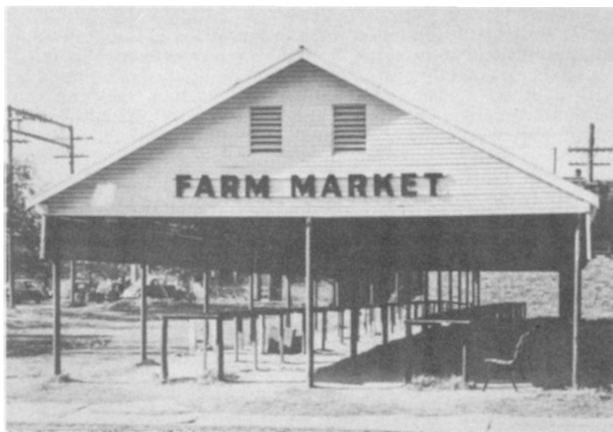
Farm market shed, Norman, Oklahoma, erected by Chamber of Commerce, Extension Division, cooperating.
