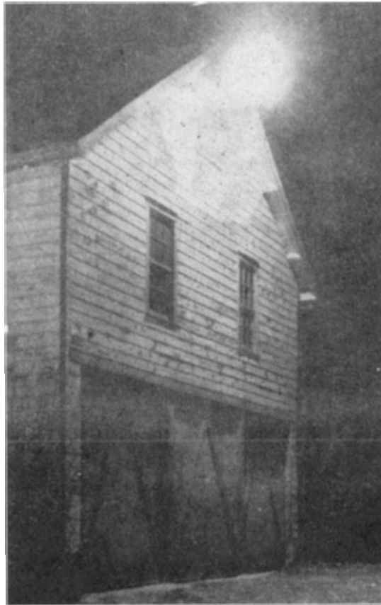
Fig. 14.—Barn yard light.
