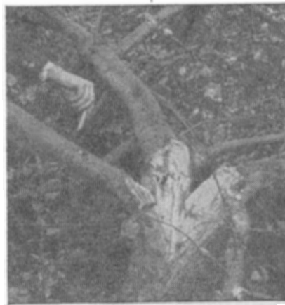
Fig. 4.—This matured apple tree was destroyed because of narrow angles between the branches and the trunk. Branches located too close together also weakened the tree.
