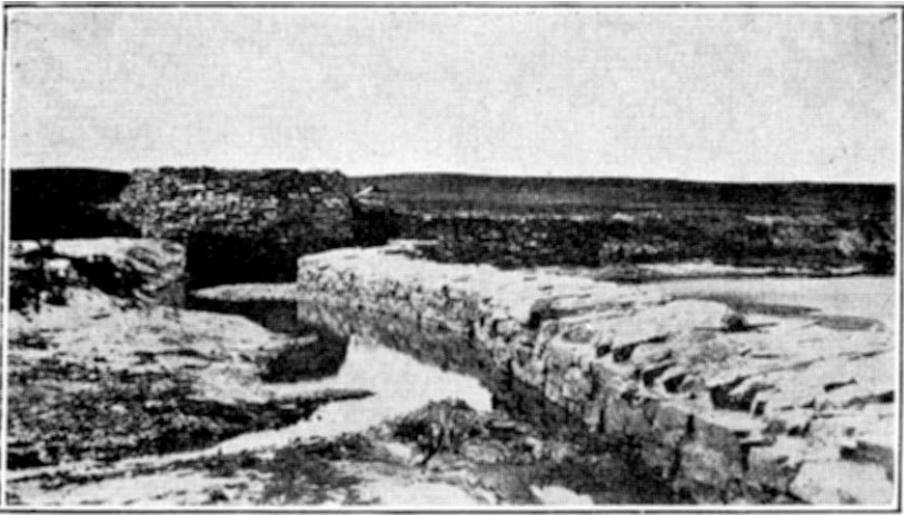
Figure 4—Rock Dam in Cimarron River
