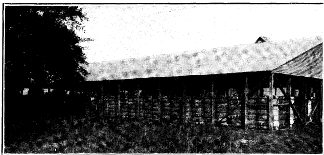
A CHEAP AND VERY SATISFACTORY COTTON WAREHOUSE Stillwater, Payne County, Oklahoma
