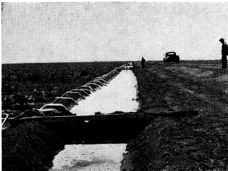
Figure 7.—Temporary canvas check and two-inch metal syphons used together for distribution of water to field.
