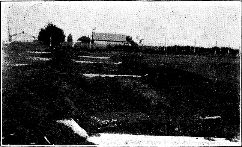
Figure 9.—The Dam Should Maintain the Shape of the Ditch.
