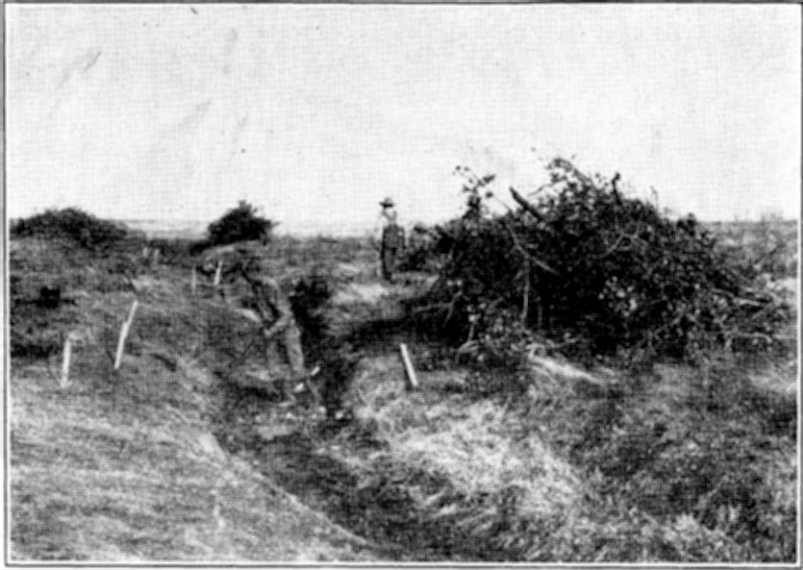
Figure 2.—Starting to Reclaim a Gully Washed Down to Bed Rock—Guthrie Project
