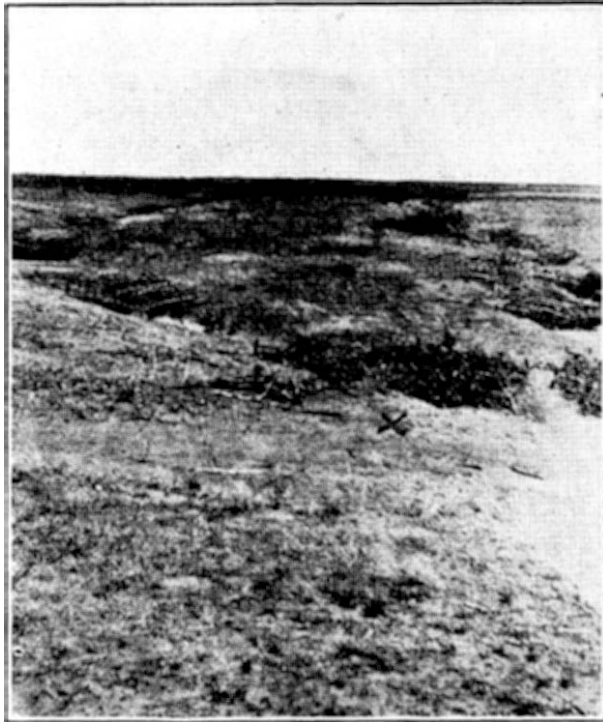
Figure 4.—Reclaiming a Hillside Field with Brush and Straw Dams.—Guthrie Project.
