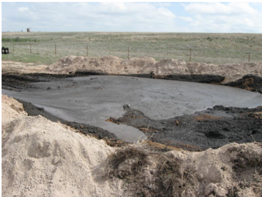
Figure 8.3. Oil-base mud shown in a staging cell constructed of gypsum, prior to mixing with gypsum and subsequent land application.
