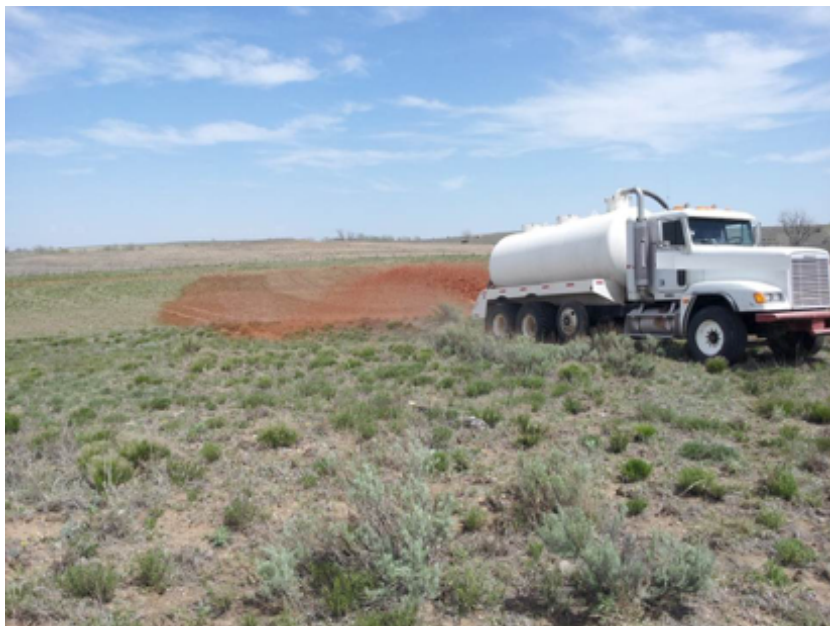
Figure 8.4. Example land application of water-base mud (WBM).
