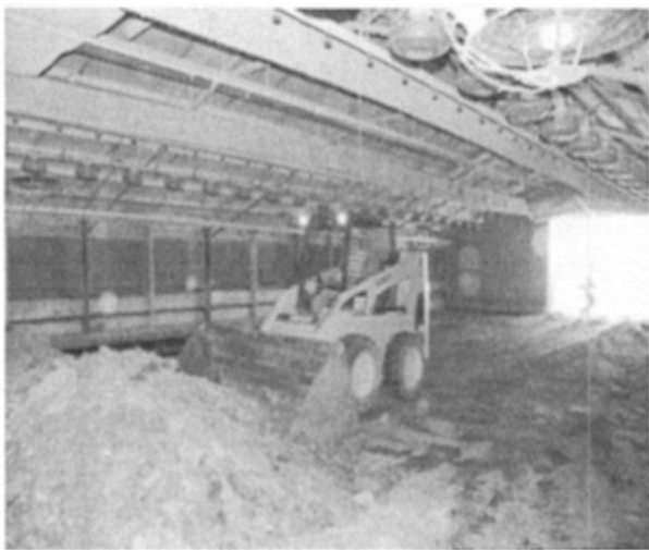
Figure 2. Poultry house during cleanout.
