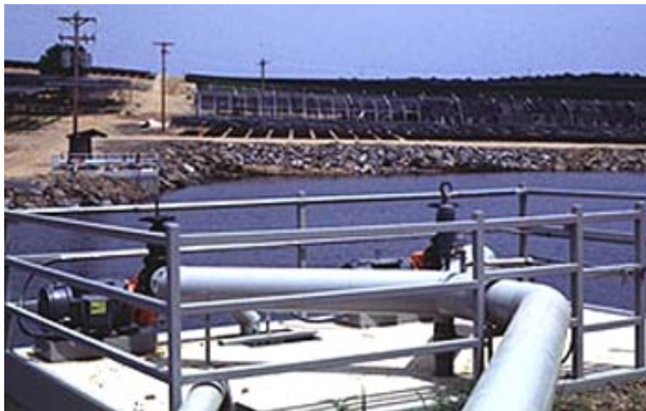
Shown here is a retention basin for capturing irrigation runoff and equipment for pumping captured water to a storage pond at a higher point in the nursery. In the storage pond, the water can be mixed with fresh water and held for later use.
