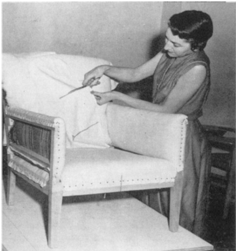
Fig. 32 Cutting Fabric to Fit Around Arm Post
