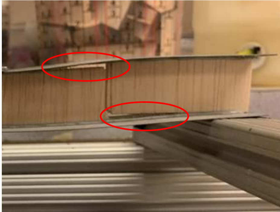
Figure 80: Inspection of Failure in 10" I-Beam
