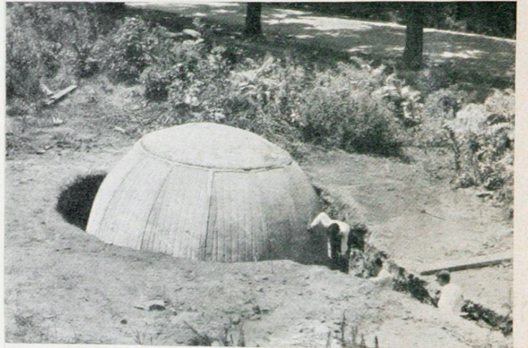
After careful study of bombs and shelters in war, Americans have designed a new concrete pillbox which can be built in five hours
