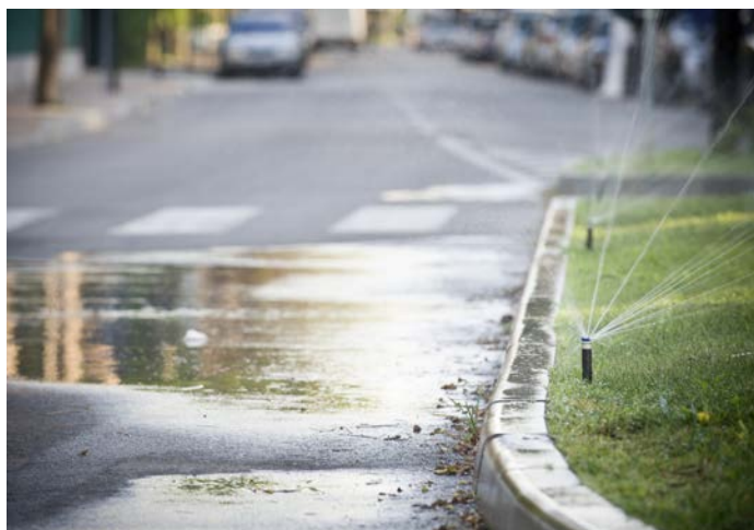
Figure 13. Check the performance of irrigation components on a regular basis. Adjust or repair as needed to prevent watering streets and driveways.
