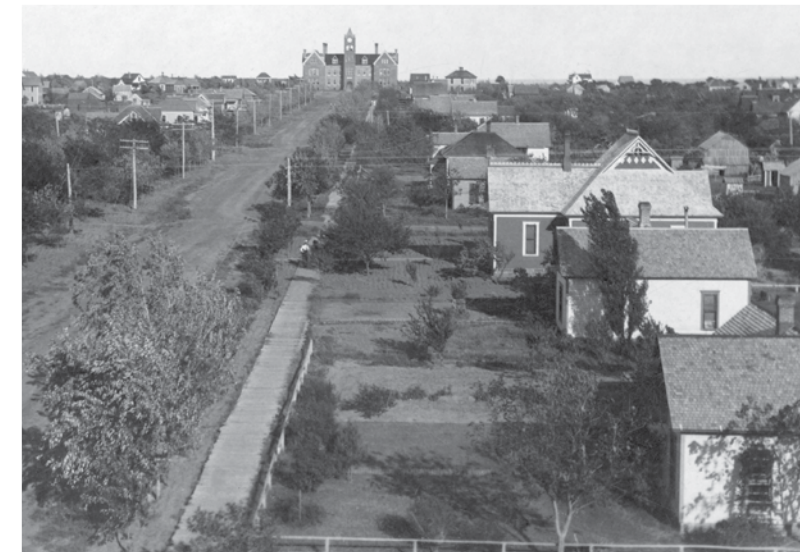
UCO's Director of Archives Nicole Willard says this is her favorite Old North photo, showing the wooden walkway that kept people out of the dirt, sometimes mud, street that led to Old North in earlier times. The back of the photo tells how walkway nails would work their way up and snag the hems of women's long dresses.
