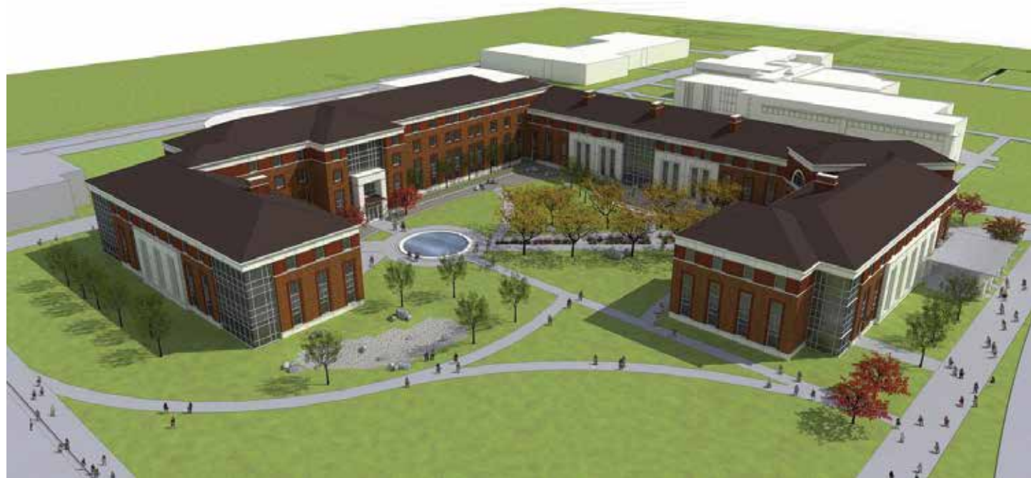
Officially being named the Transformative Learning Quadrangle, the new residence hall has already been dubbed 'The Quad.' While offering 440 new beds, the structure also will offer common living and study areas, even for non-resident students.
