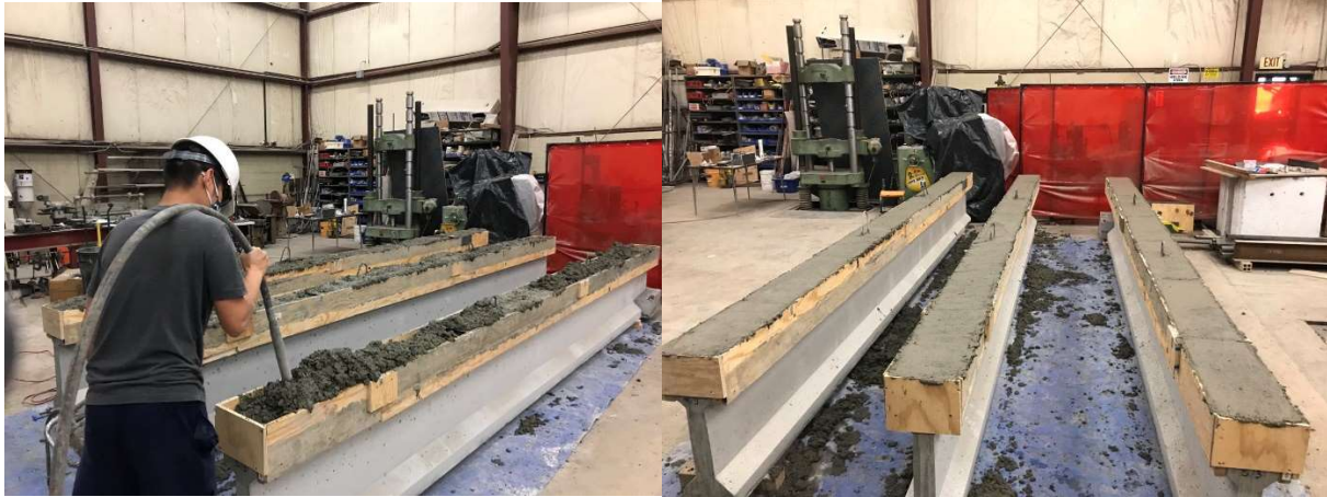
Figure 3.9: Casting Deck (Left) and Finishing Deck Casting (Right)
