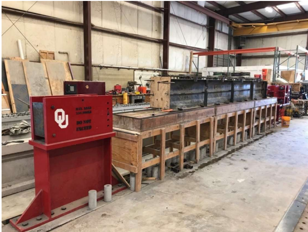
Figure 3.6: Prepared Formwork for Casting
