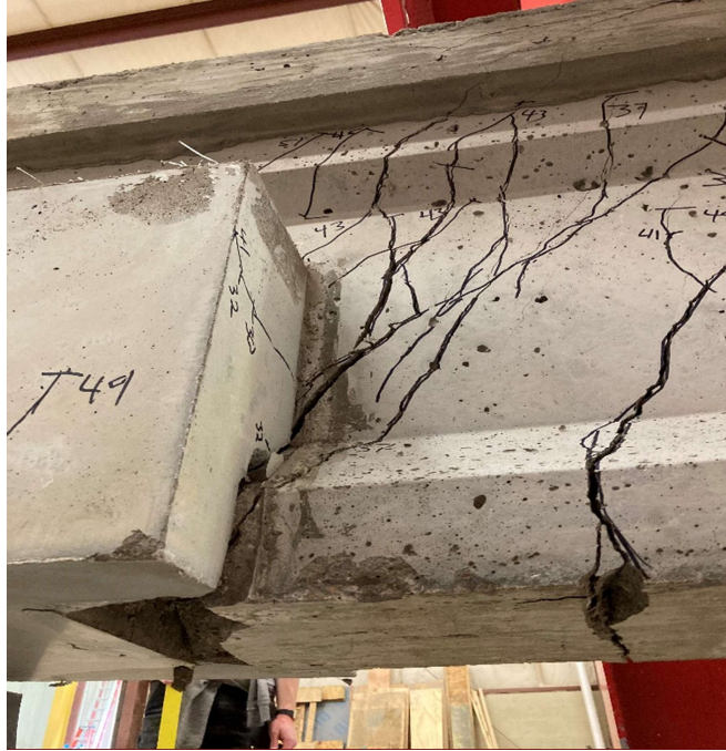
Figure 4.14: Cracks in Bottom Flange of FR-SCC-1 Girder after Test
