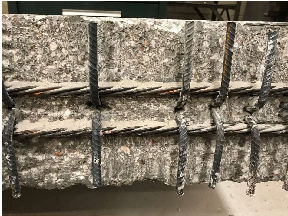
Figure 3.11: Surface Preparation at the Corroded Region
