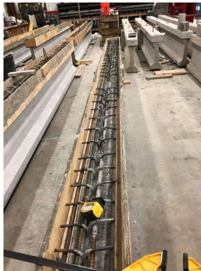
Figure 3.8: Deck Formwork Preparation
