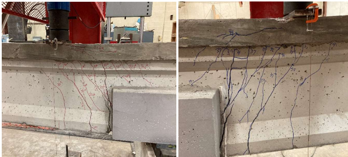
Figure 4.6: MALP-2 Girder after Test with SW Side (Left) and SE Side (Right)
