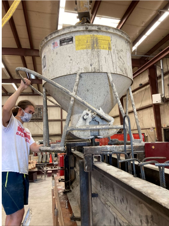
Figure 3.7: Casting Girder without Vibration
