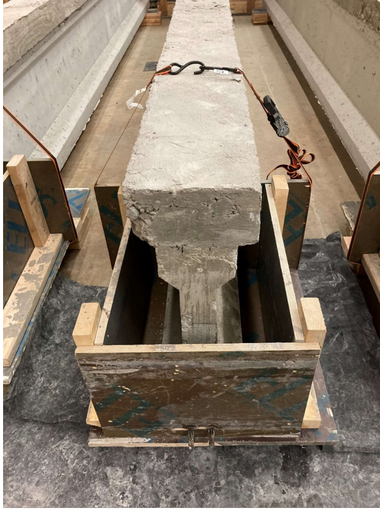
Figure 3.12: Formwork Encapsulating the Repaired Region
