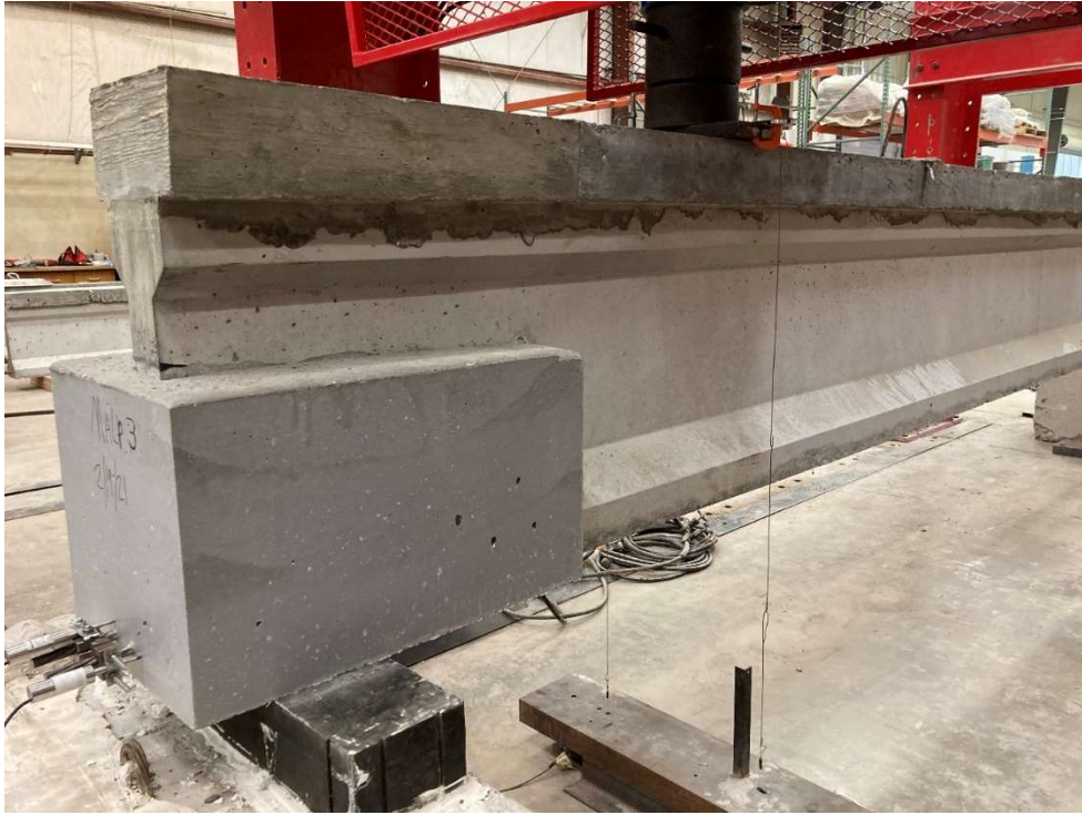
Figure 3.22: Finished MALP Repaired Girder
