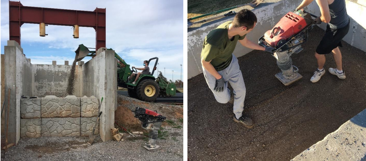
Figure 9 – Filling and compacting the abutment model; (Left) dumping aggregate via front-loading tractor; (Right) compaction pattern
