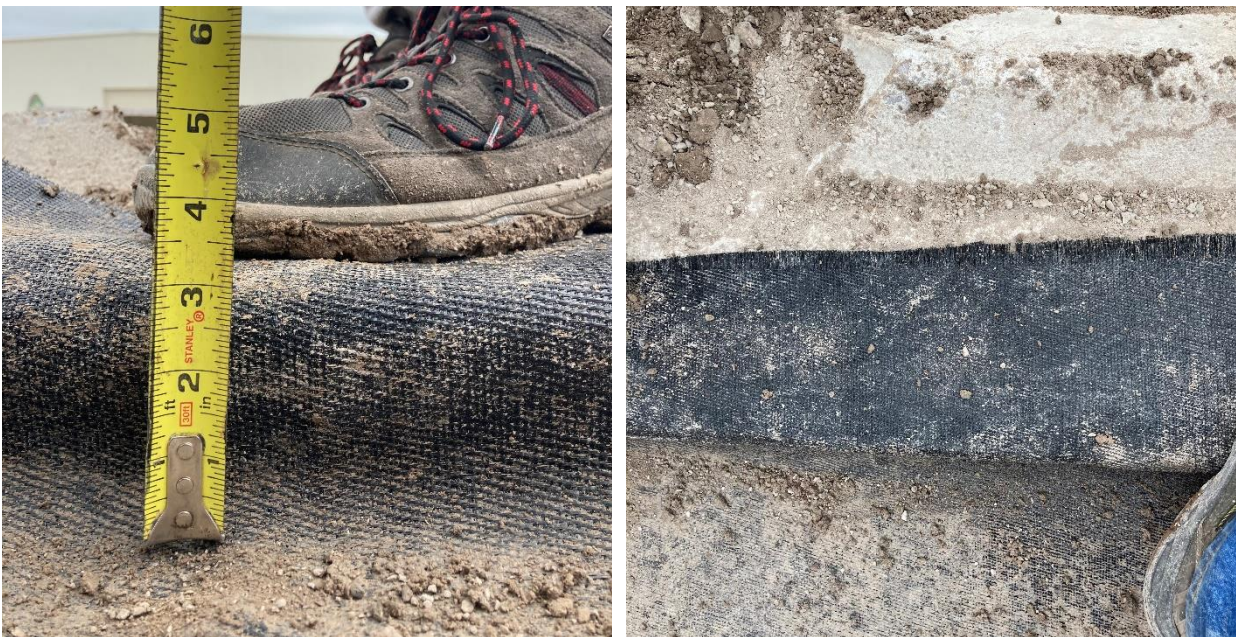
Figure 25 – Reinforcement at 75-inch elevation of GRS Abutment Model #7
