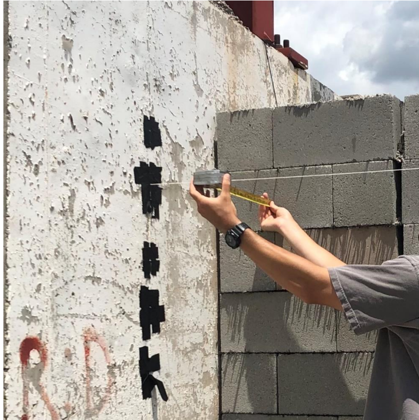
Figure 11 – Facing deformation survey measurement
