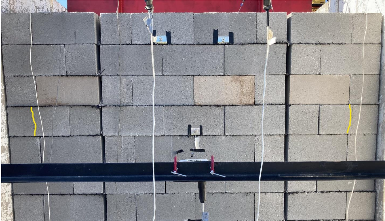
Figure 34 – CMU fractures from GRS Abutment Model #8 performance test (outlined in yellow)
