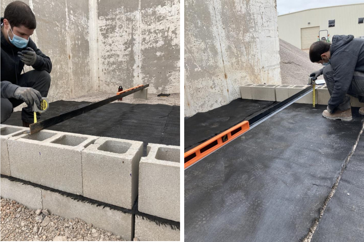
Figure 12 – Elevation survey measurement
