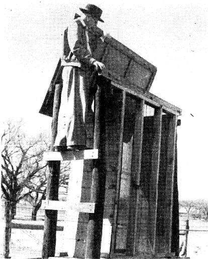
Figure 13. Column driers were constructed for loading from top.
