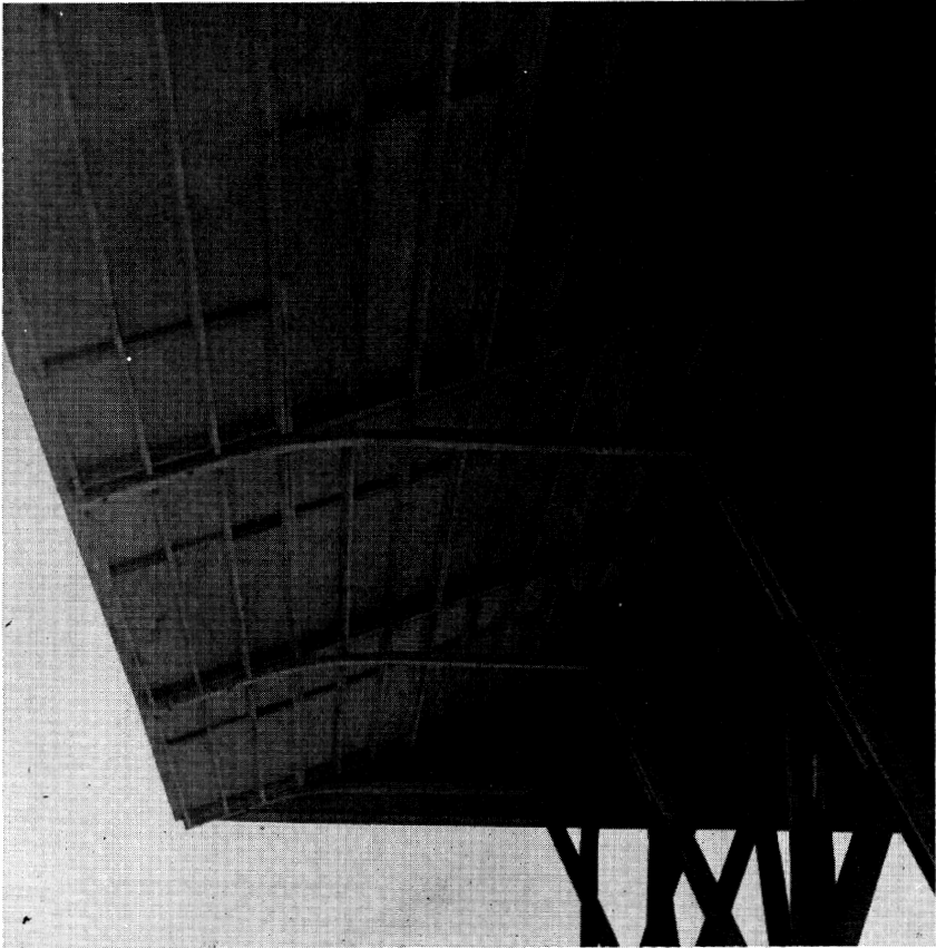
Figure 6. Hay storage erected with 4 ft. by 12 ft. plywood stressed-skin panels on glue-laminated umbrella-type frame supported by pole bipods.
