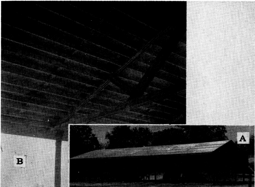
Figure 5. Shelter building erected with 4 ft. by 12 ft. plywood stressed-skin panels on sandwich trusses. (A) Exterior appearance (B) Appearance under the roof.
