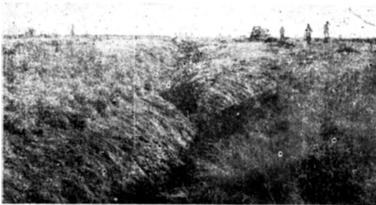
Figure 11. A gully on the East Farm at the Red Plains Conservation Experiment Station after the banks had been sloped and prepared for construction of vegetative dams and revegetation.
