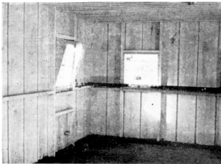
Interior view of 12x16 ft. stationary straw-loft brooder house showing door in north side opened, window and chick exit door on west side, framing and construction, and ceiling for straw loft.
