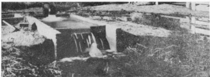
Water is pumped from an irrigation well into a concrete box equipped with gates to direct the flow into different head ditches.
