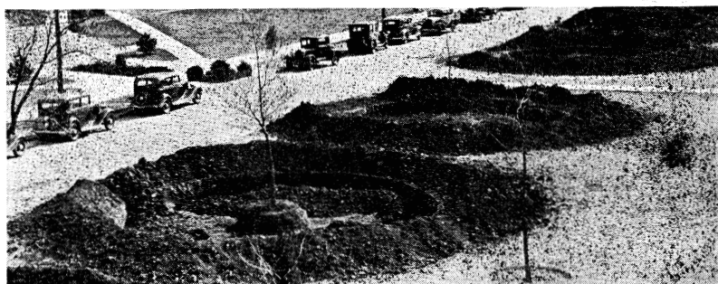
Figure 6. Soil removed from pits thirty feet in diameter surrounding young trees in order to modify a dense clay subsoil by the addition of very fine sand. Thirty tons of very fine sand were mixed in each of these pits and an equivalent amount of dense clay was discarded.
