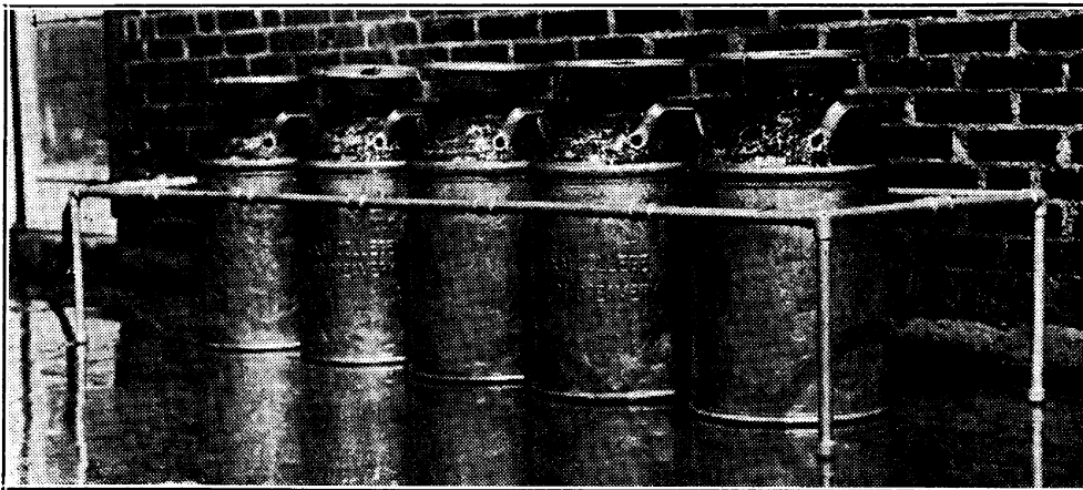
Figure 10. An evaporation cooler recommended for use in cream station.
