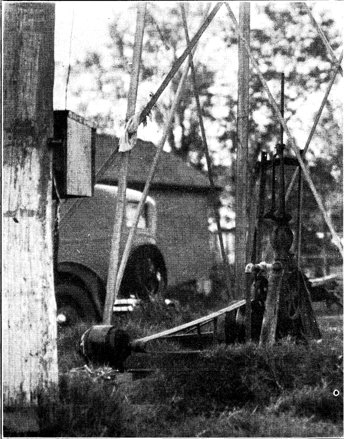
Mr. C. R. Birks' damaged windmill was replaced with an electric motor and pump jack. The motor is kept covered for protection from the weather.
