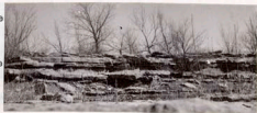
Figure 9. Middle spillway at Phillip's Lake, N.W. \frac{1}{4} sec. 10, T. 26 N., R. 6 E. Hughes Creek limestone beds below the chert zone.
