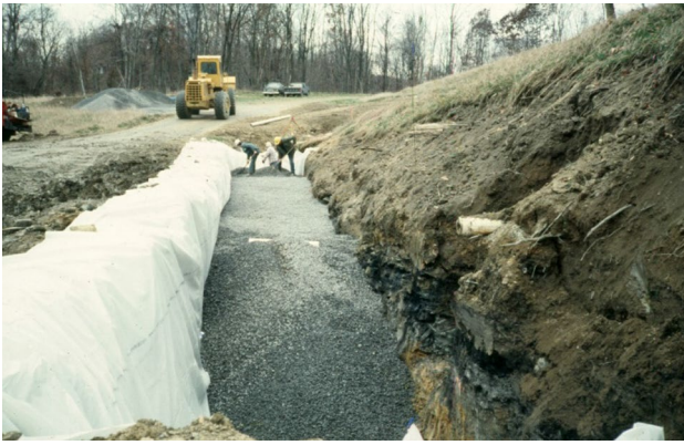
Fig. 5 An anoxic limestone channel being constructed, soon to be covered with the plastic sheeting and a soil cover
