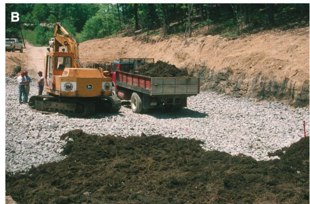
Fig. 5 An anoxic limestone channel being constructed, soon to be covered with the plastic sheeting and a soil cover
