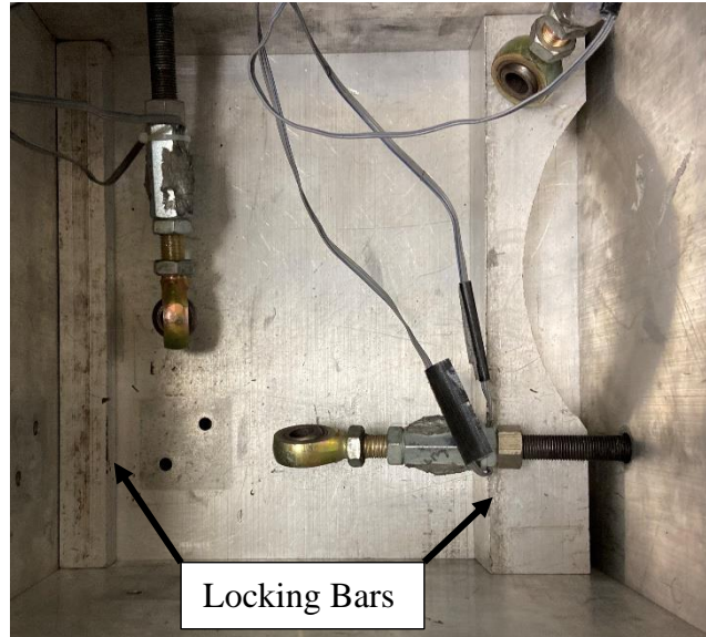
Figure 4.32 – Locking bars placed to reduce movement of inset plates
