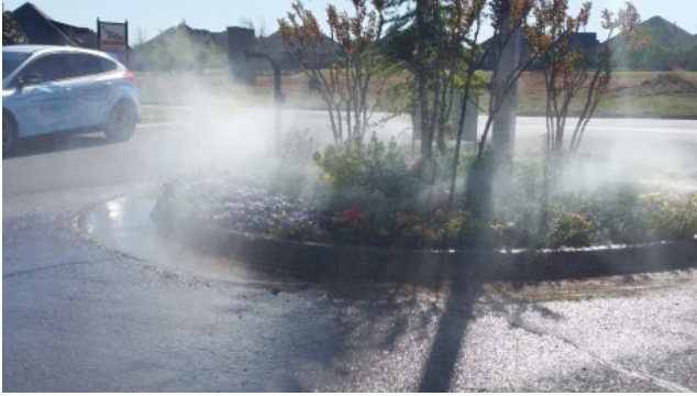
Figure 2. Example of extremely high pressure resulting in misting. (photo courtesy of Joshua Campbell, Oklahoma State University)
