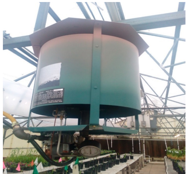
Figure 3. Carbon dioxide generator manufactured by Johnson Gas Appliance Company (Iowa). The generator operates with either propane or natural gas and has pressure gauge to control the size of burner.
