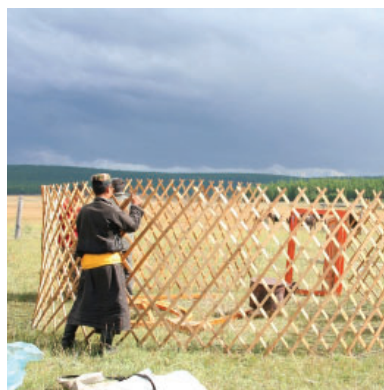
Picture (10) Finished frame of yurt in Kazakhstan, before covering it with carpets or fabric.
