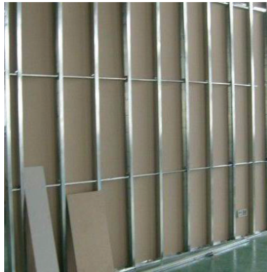
Picture (28), (29) Examples of construction process of the gypsum plasterboard partition wall. Frame structure
