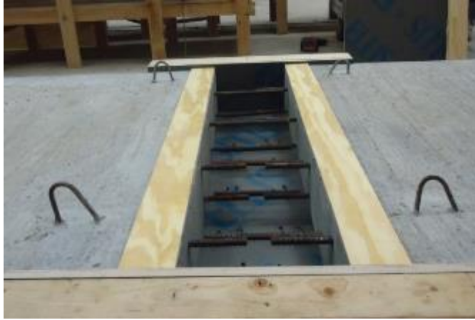
Figure 82. UHPC slab joint formwork and reinforcement before placing the formwork top
