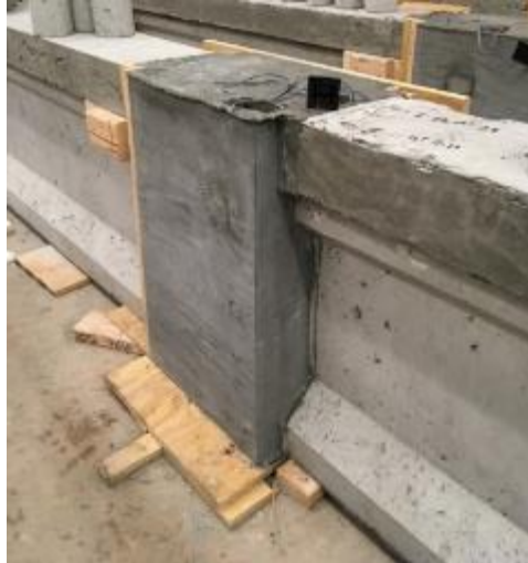
Figure187. Completed continuity joint representing retrofit of an existing structure
