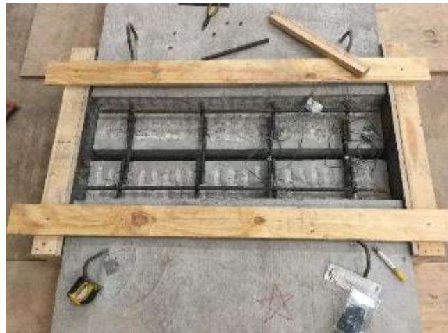
Figure 991. Two slab panels with formwork in place and strain gauges installed
