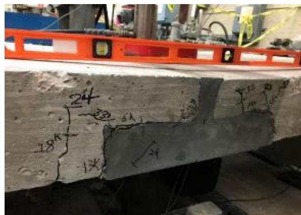
Figure 126. Cracks formed at interface between UHPC and conventional concrete and underneath the load point on the south side of J3 slab joint 1
