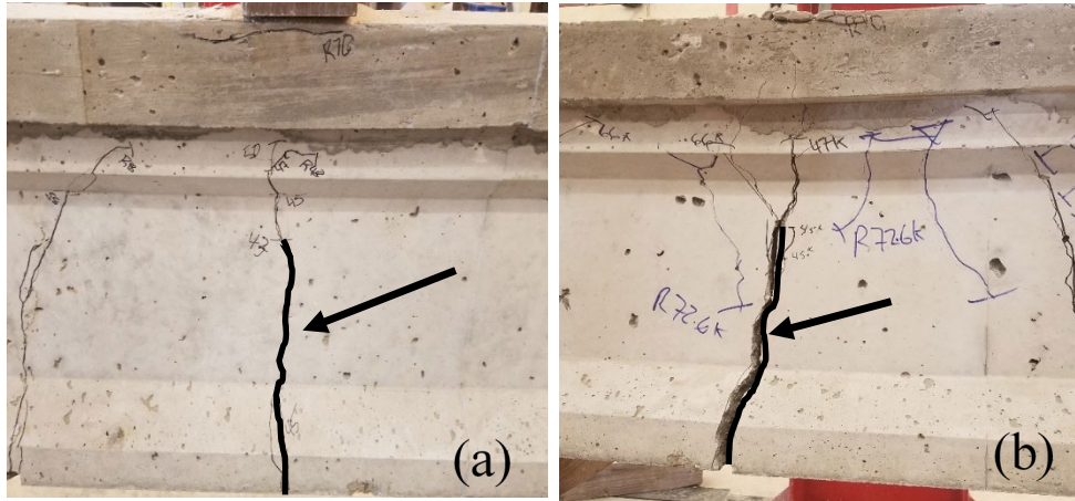
Figure 196. Initial flexural cracking under the load point on the NC1-N girder at 43 kips of load (a) and initial flexural cracking under the load point on the NC1-S girder at 45 kips of load (b). Arrows point to the dark lines that indicate the initial flexural cracks.
