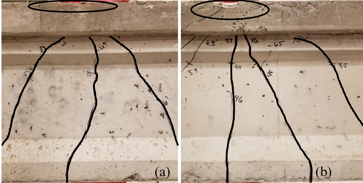
Figure 254. Final flexural cracking under the load point in the RC3-N (a) and RC3-S (b) girders are indicated by dark lines and concrete deck crushing is indicated by dark ovals.
