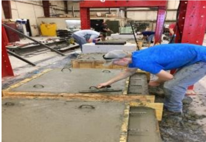
Figure 93. Finishing the top surface of the base concrete slabs
