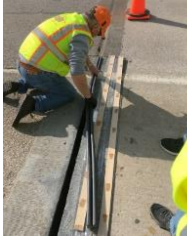
Figure 334. Installation of joint sealant material by SSI Highway Products personnel
