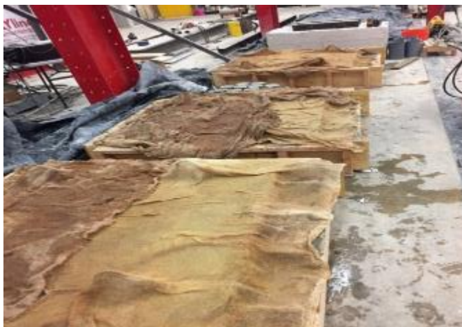
Figure 95. Concrete slabs curing covered by wet burlap
