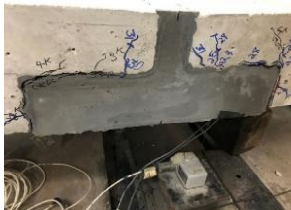
Figure 136. Cracks formed at the conventional concrete to UHPC interface and propagating upward on the south side of J3 slab joint 2
