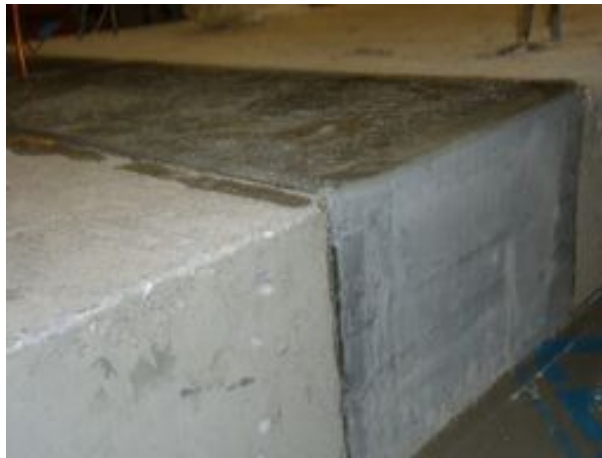
Figure 86. Completed Ductal® slab joint after formwork removal
