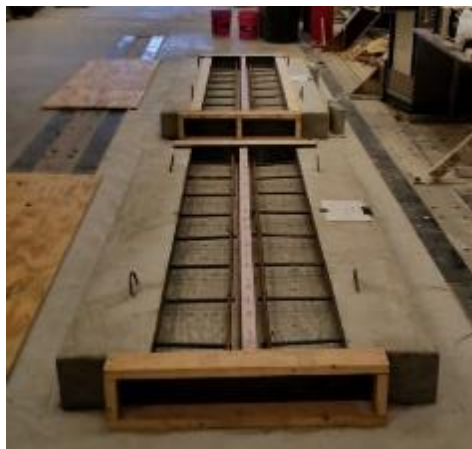
Figure 340. Demonstration joint specimens before UHPC placement
