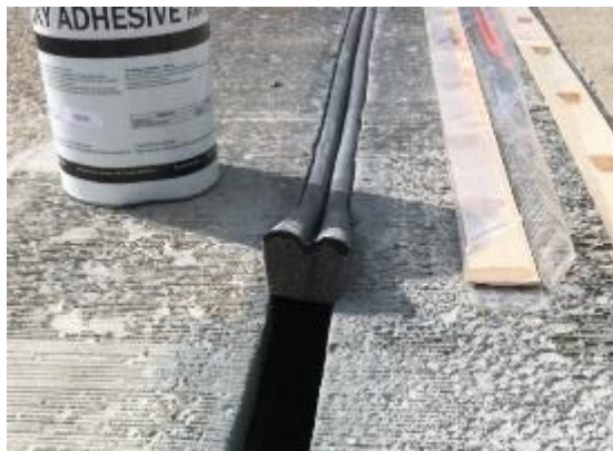
Figure 335. End of joint sealant prepared for splicing
