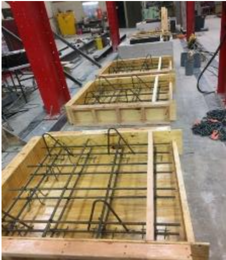
Figure 89. Formwork prepared for concrete casting
