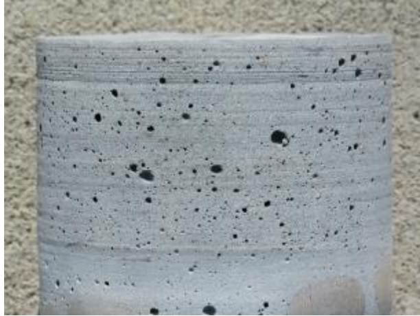
Figure 119. Non-proprietary UHPC slab joint core indicating uniform consistency
