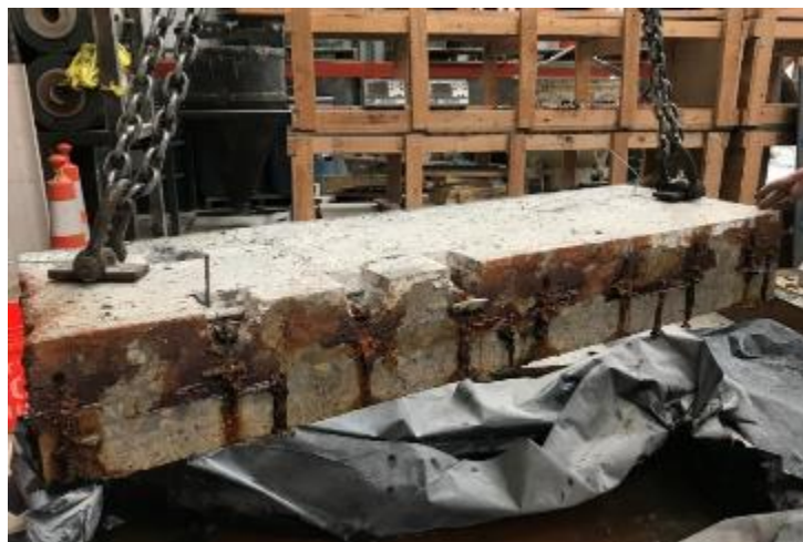
Figure 311. Typical level of reinforcing bar corrosion at the conclusion of testing - week 10
