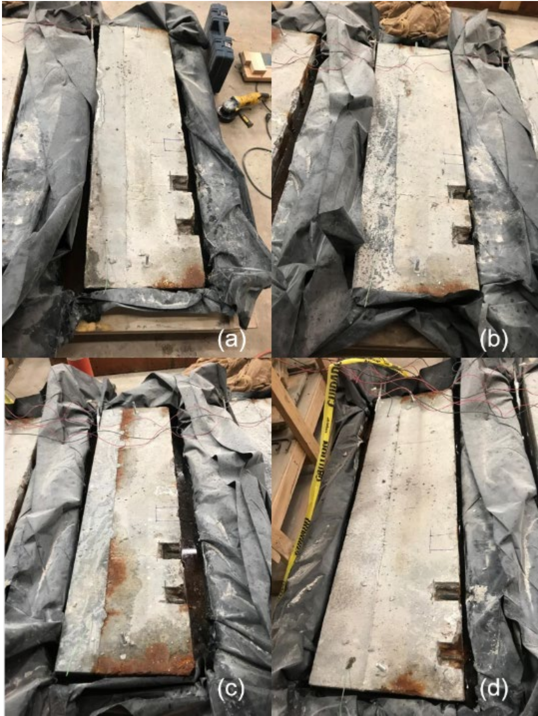
Figure 315. Week 6 update for large-scale corrosion specimens using (a) ODOT AA, (b) J3, (c) Ductal®, and (d) Phoscrete
