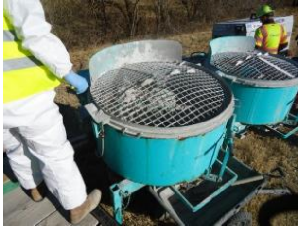
Figure 329. High shear mixers used for mixing UHPC
