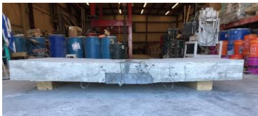
Figure 129. J3 Slab joint 1 curvature after failure
