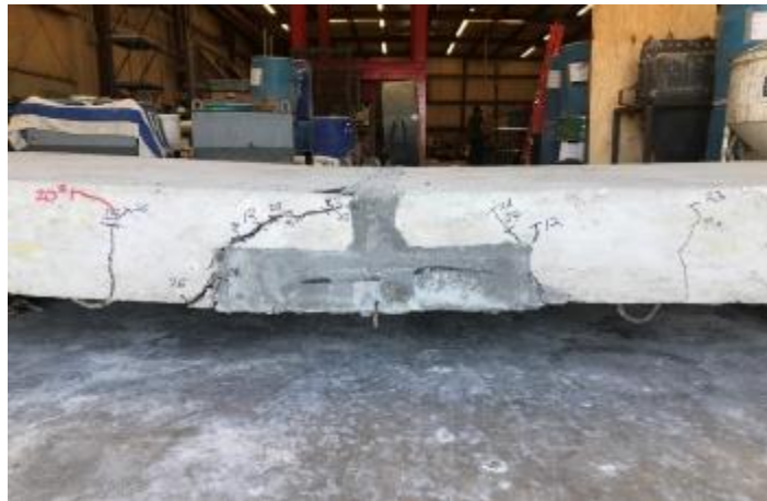
Figure 143. Ductal® slab 1 after part 2 of testing
