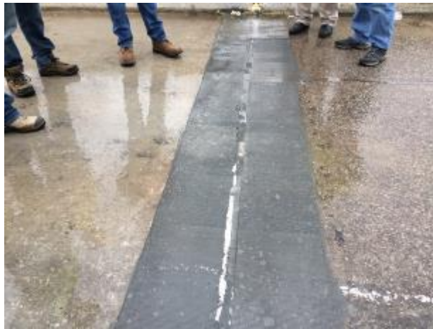
Figure 333. Entire joint after grinding
