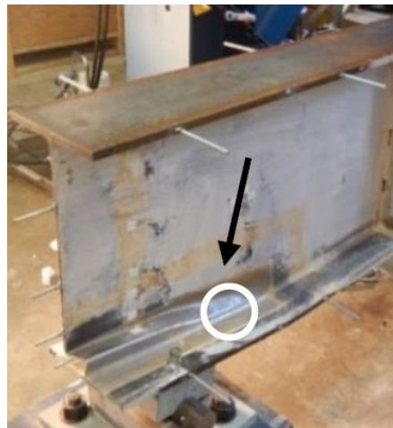
Figure 14. Damaged girder failure (Zmetra 2015)
