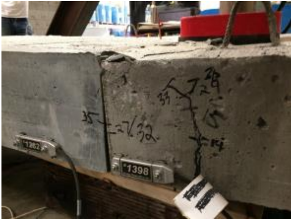
Figure 109. Cracking near the load point at failure for Ductal® slab joint 2
