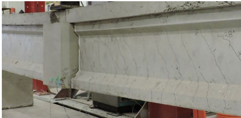
Figure 4.108. Specimen R1-FRSCC shear and flexural cracking
