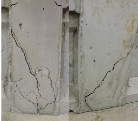
Figure 4.76. Initial cracking of specimen R2-PHOS on the front (left) and rear (right) of the joint face
