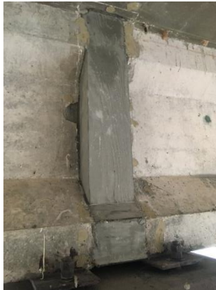
Figure 7.30. Completed UHPC continuity joint after form removal
