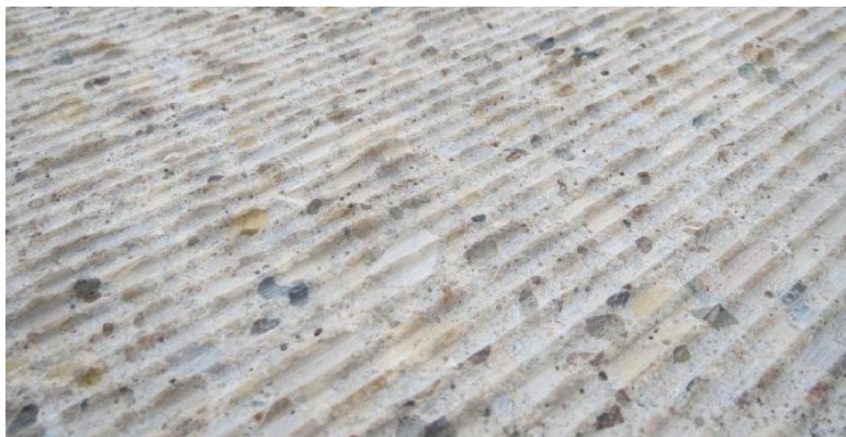
Figure 2.6. Final bridge deck substrate preparation (Graybeal 2017)
