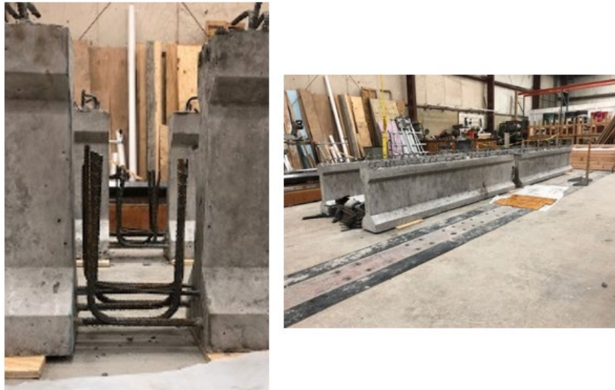
Figure 4.23. Orientation of half-length girders prior to deck/joint casting
