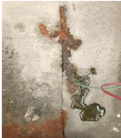
Figure 6.21. Green liquid in joint of Phoscrete® large-scale corrosion specimen during week 10 of testing
