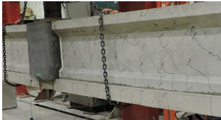
Figure 4.95. Specimen R2-J3 shear and flexural cracking
