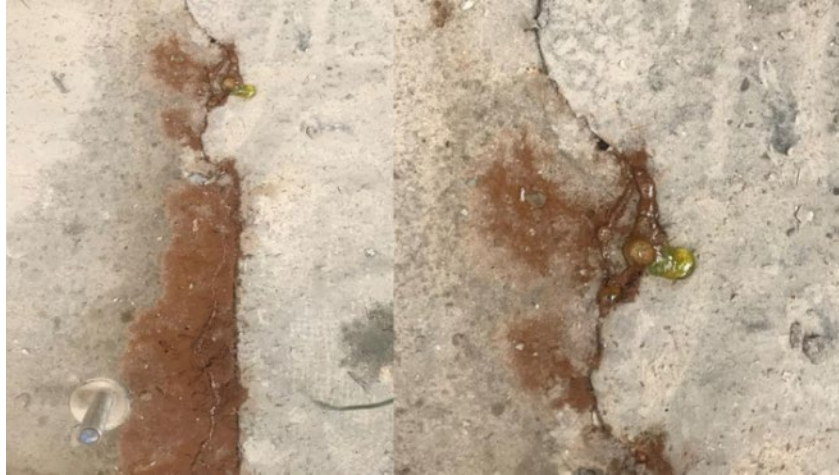
Figure 6.20. Green liquid in joint of Ductal® large-scale corrosion specimen during week 8 of testing
