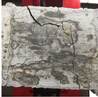
Figure 4.79. Initial cracking of specimen R3-PHOS on the bottom joint face
