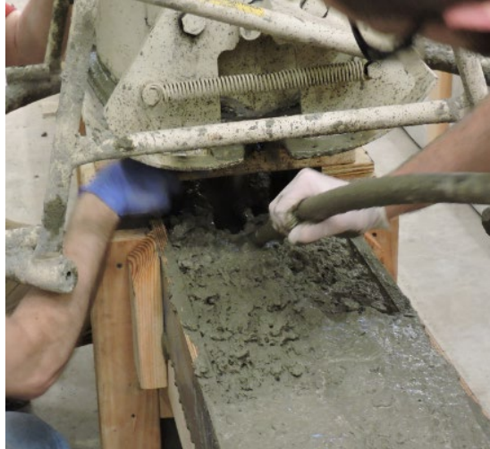
Figure 4.32. Vibrating the continuity joint during casting
