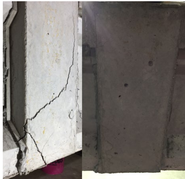
Figure 4.68. Initial cracking of specimen R1-FRSCC on the front (left) and rear (right) of the joint face
