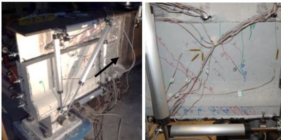
Figure 2.18. Repaired girder failure (Zmetra 2015)
