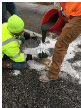
Figure 7.27. Placement of UHPC into fill hole in the bridge deck
