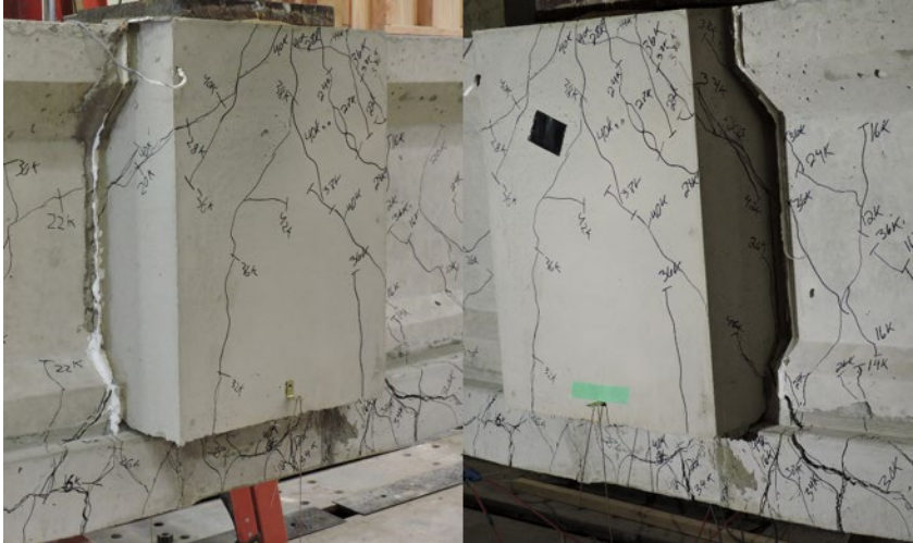
Figure 4.121. Specimen R3-FRSCC joint cracking on the longitudinal and transverse faces from the front left (left) and front right (right)
