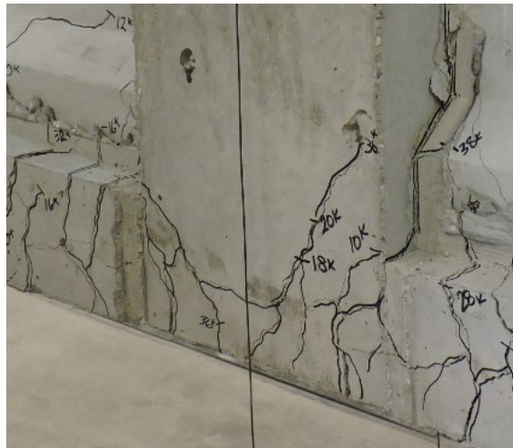
Figure 4.47. Specimen C2 flexural cracking in the continuity joint
