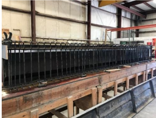
Figure 5.5. Reinforcement cage for a typical girder
