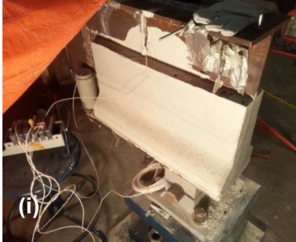
Figure 2.15. Final repaired girder (Zmetra 2015)
