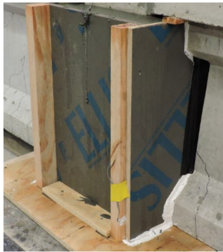
Figure 4.88. Joint repair formwork
