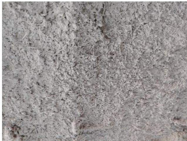
Figure 7.8. Close-up of MALP repair after placement of the first layer
