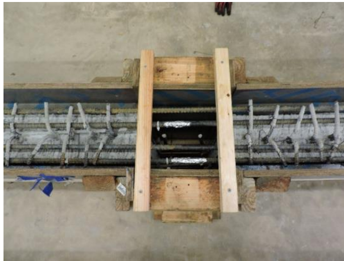
Figure 4.29. Top view of continuity joint prior to casting
