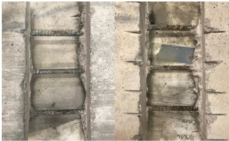
Figure 6.8. Corrosion state of rebar reinforcing at joint of Phoscrete® small-scale corrosion specimens with 4% NaCl (left) and 8% NaCl (right)
