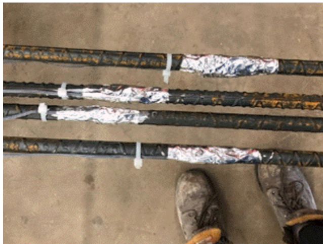
Figure 4.28. Strain gauges attached to longitudinal reinforcement ready for installation
