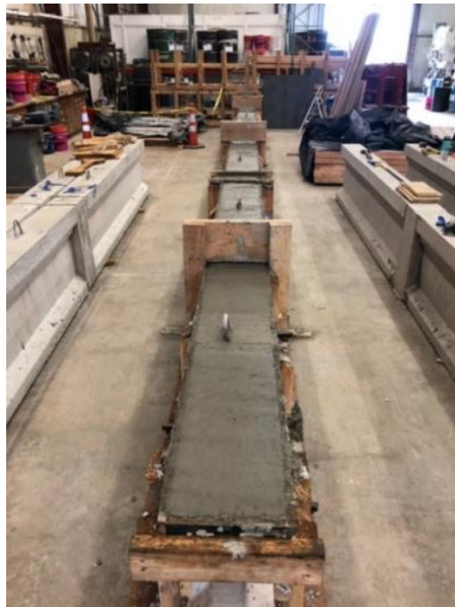
Figure 4.33. Girder-joint-girder specimen after final casting
