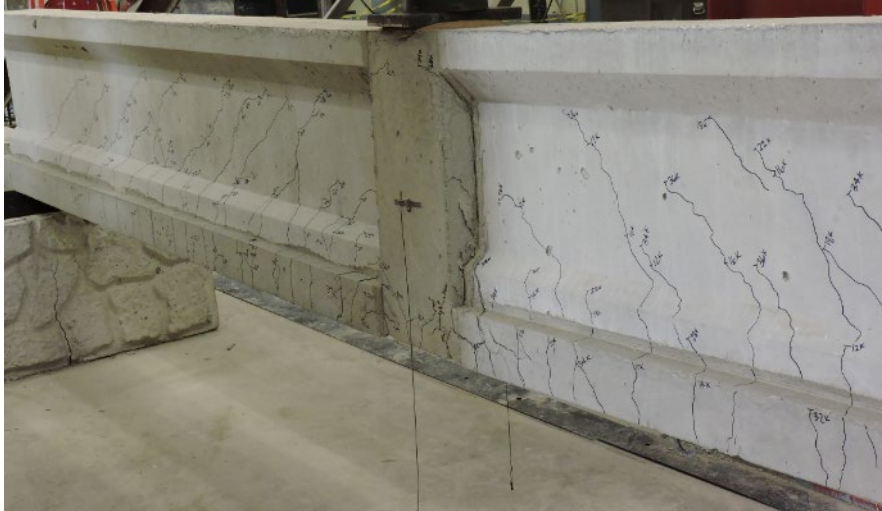
Figure 4.38. Specimen C1 shear cracking
