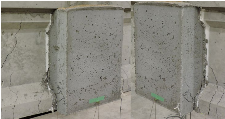
Figure 4.127. Specimen R1-PHOS girder-joint interface and joint transverse face cracking from the front left (left) and front right (right)
