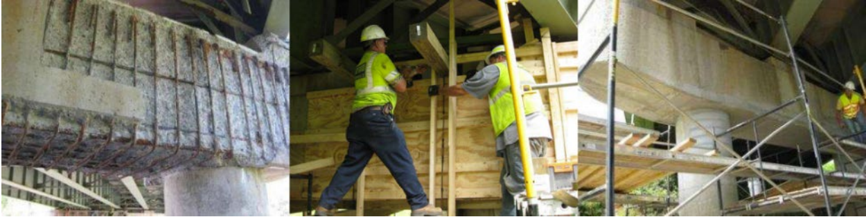
Figure 2.30. SCC repaired column and pier cap (Ozyildirim 2013)
