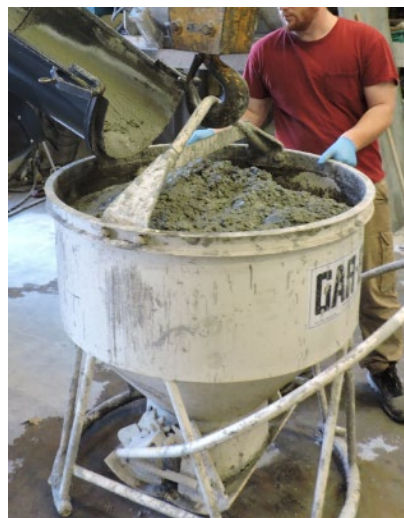
Figure 4.19. Filling round-gate bucket with concrete
