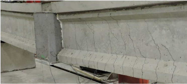
Figure 4.126. Specimen R1-PHOS shear and flexural cracking
