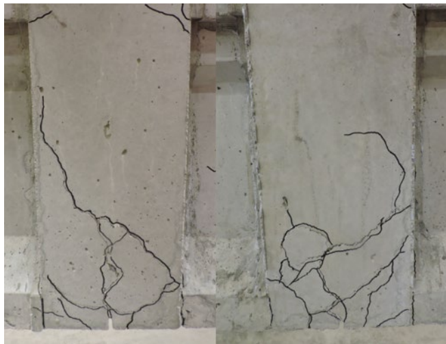
Figure 4.66. Initial cracking of specimen R3-J3 on the front (left) and rear (right) of the joint face
