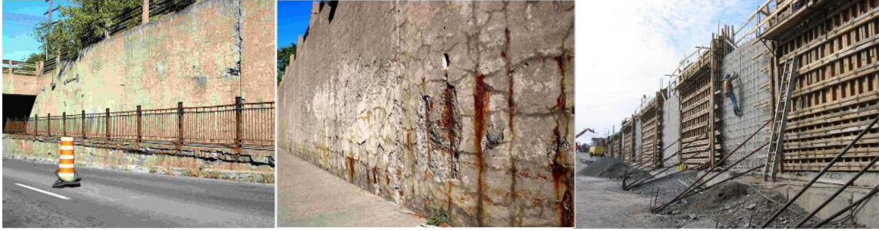
Figure 2.33. Application of FR-SCC in Jarry/Querbes underpass, Montreal (Khayat et al. 2005)
