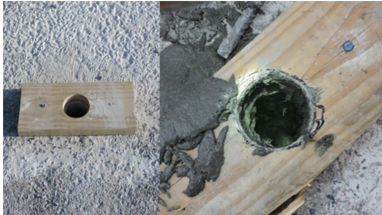
Figure 7.26. Pour holes for UHPC joints on the Wolf Creek bridge
