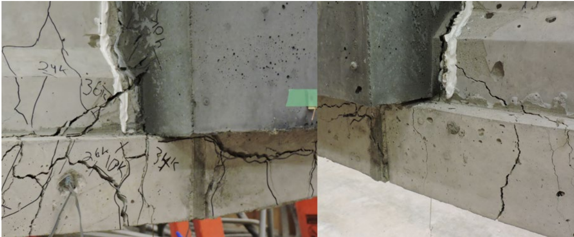
Figure 4.97. Specimen R2-J3 girder-joint interface cracking on the front left (left) and front right (right)
