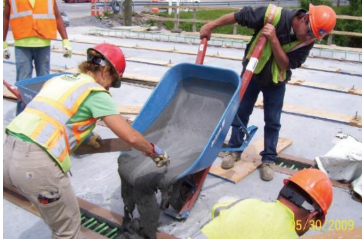
Figure 2.5. UHPC placement into a longitudinal connection of bridge elements (Graybeal 2014)
