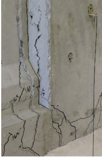
Figure 4.48. Specimen C2 cracking at girder-joint interface (left side)
