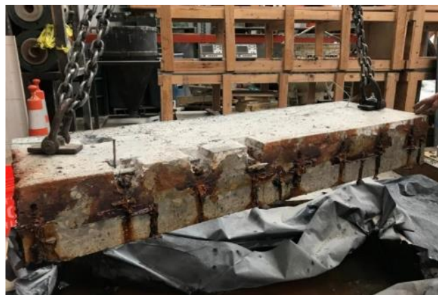
Figure 6.24. Typical reinforcing bar corrosion at the conclusion of testing - week 10
