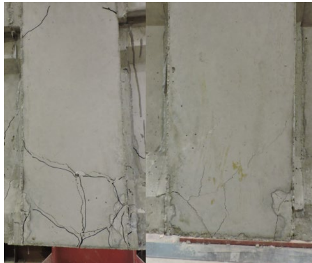
Figure 4.70. Initial cracking of specimen R2-FRSCC on the front (left) and rear (right) of the joint face
