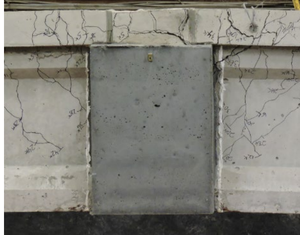
Figure 4.96. Specimen R2-J3 continuity joint repair after testing
