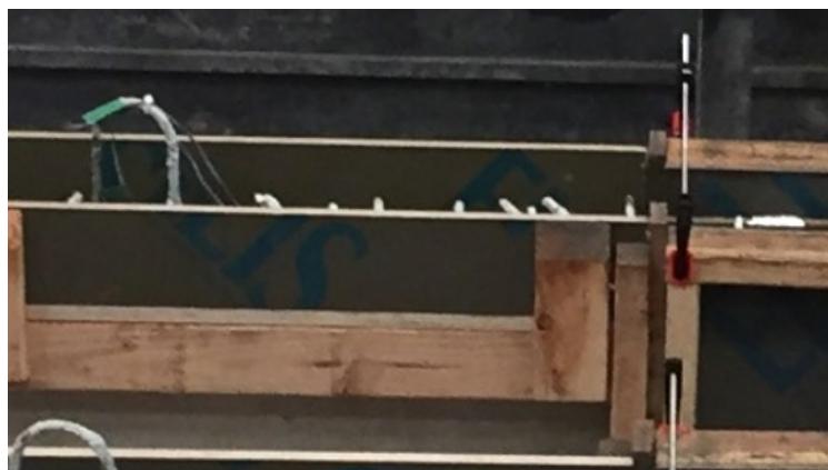
Figure 4.30. Strain gauge wires before casting the continuity joint and deck
