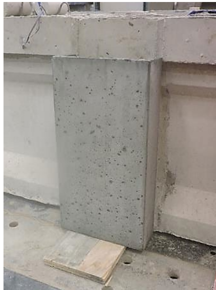
Figure 3.30. J3 UHPC continuity joint repair mock-up specimen
