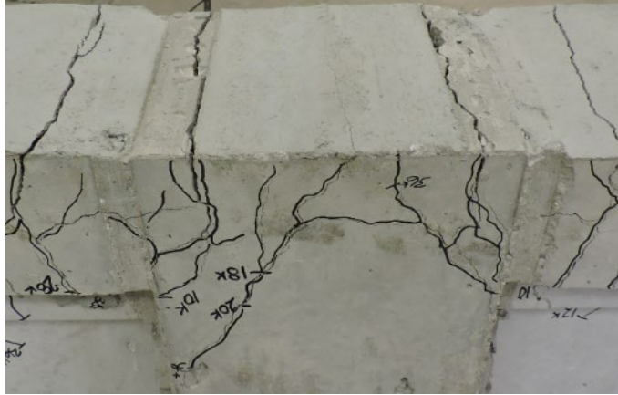
Figure 4.50. Specimen C2 girder-joint interface cracking across the deck
