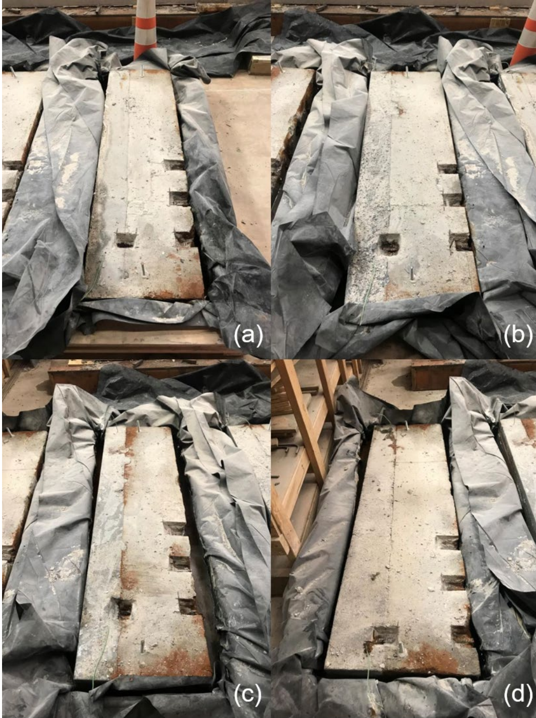
Figure 6.29. Week 10 update for large-scale corrosion specimens using (a) ODOT AA, (b) J3, (c) Ductal®, and (d) Phoscrete®
