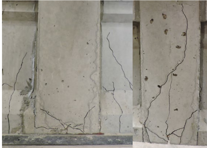
Figure 4.62. Initial cracking of specimen R1-J3 on the front (left) and rear (right) of the joint face
