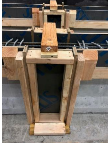
Figure 4.24. Continuity joint formwork
