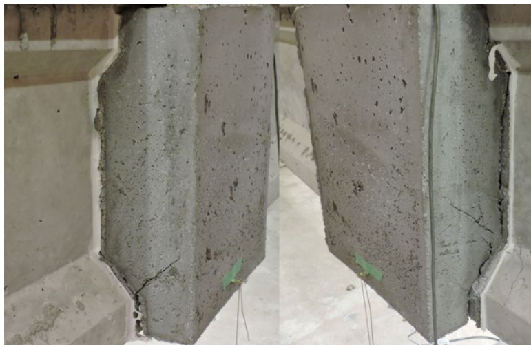
Figure 4.128. Specimen R1-PHOS girder-joint interface and joint transverse face cracking from the back left (left) and back right (right)
