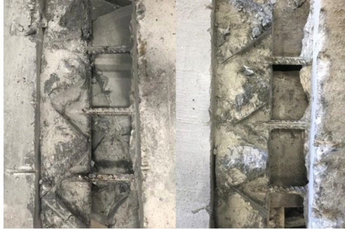
Figure 6.7. Corrosion state of rebar reinforcing at joint of Ductal® small-scale corrosion specimens with 4% NaCl (left) and 8% NaCl (right)
