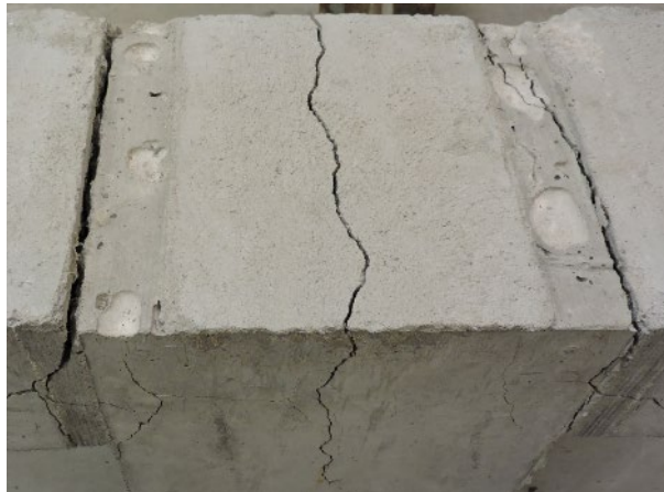
Figure 4.56. Specimen C3 girder-joint interface and centerline cracking across the deck
