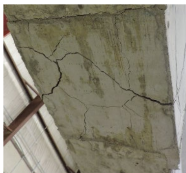
Figure 4.71. Initial cracking of specimen R2-FRSCC on the bottom joint face
