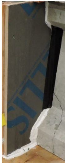
Figure 4.87. Repair formwork for side face of the continuity joint
