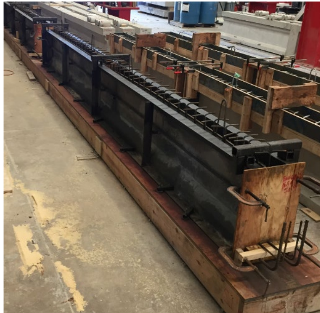
Figure 4.18. Specimen forms ready for concrete placement
