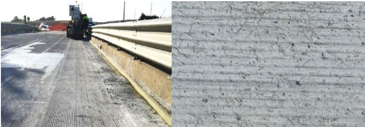
Figure 2.9. Finished overlay on the Mud Creek bridge (Wibowo and Sritharan 2018)
