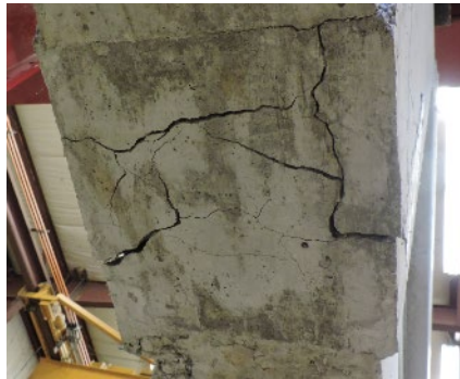
Figure 4.77. Initial cracking of specimen R2-PHOS on the bottom joint face
