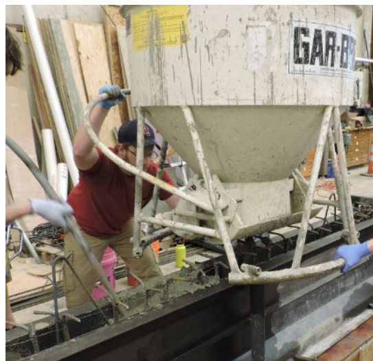
Figure 4.20. Pouring and vibrating concrete in girder formwork
