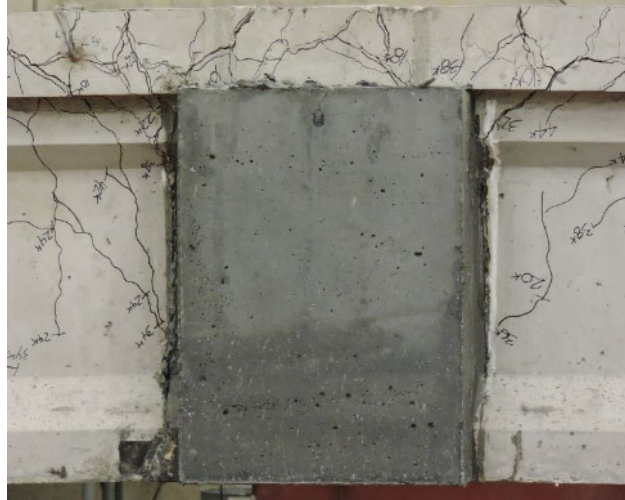
Figure 4.103. Specimen R3-J3 continuity joint repair after testing
