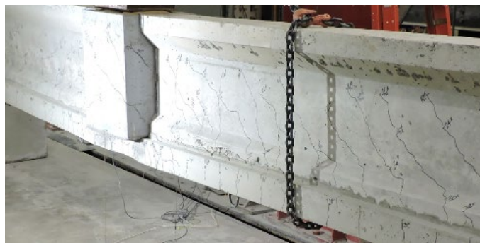
Figure 4.133. Specimen R2-PHOS shear and flexural cracking
