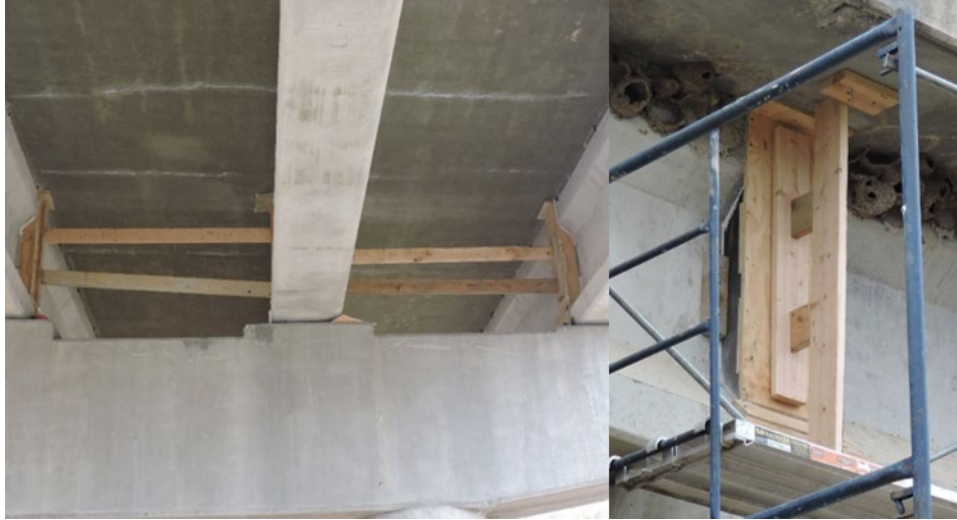
Figure 7.29. Final joint forms after adding bracing
