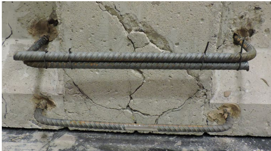
Figure 4.84. Installation of repair reinforcement
