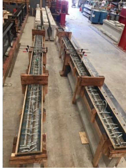
Figure 4.31. Two girder-joint-girder specimens prior to casting
