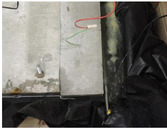
Figure 6.15. White film in water of Phoscrete large-scale corrosion specimen
