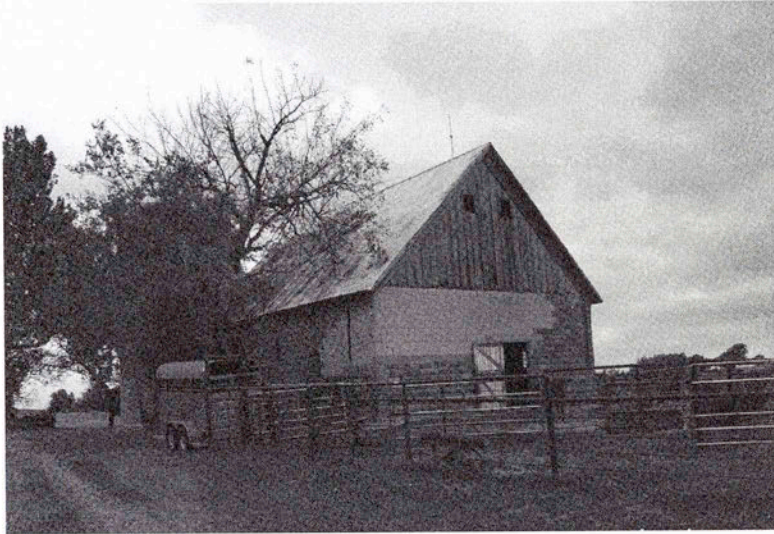
North gable end of the Samuel Graham barn built ca. 1900.
