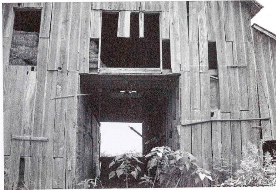
West gable end of barn with central drive through and hay loft above.
