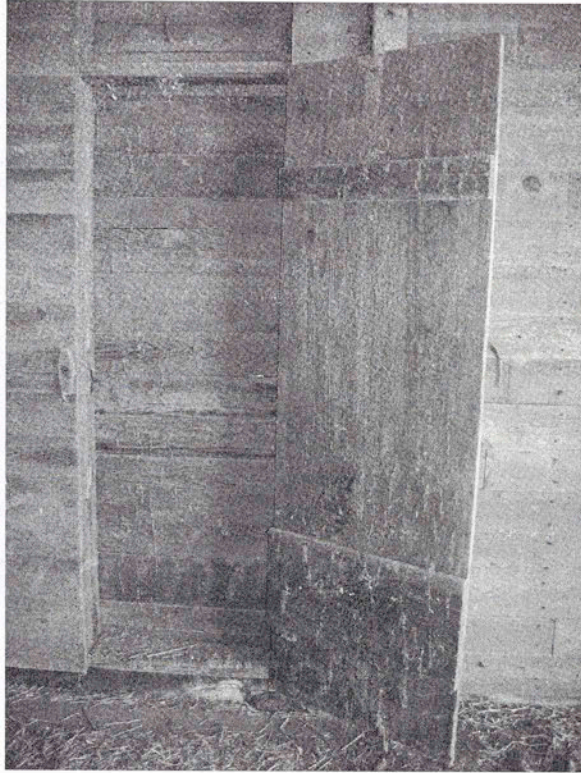
Fig. 5.4 Boards are individually removed from wooden slots located behind the door. As grain reaches various levels inside the grain bin, the boards are removed. Ralph and Alice McKeever barn (Photo by Lynda Ramsey)
