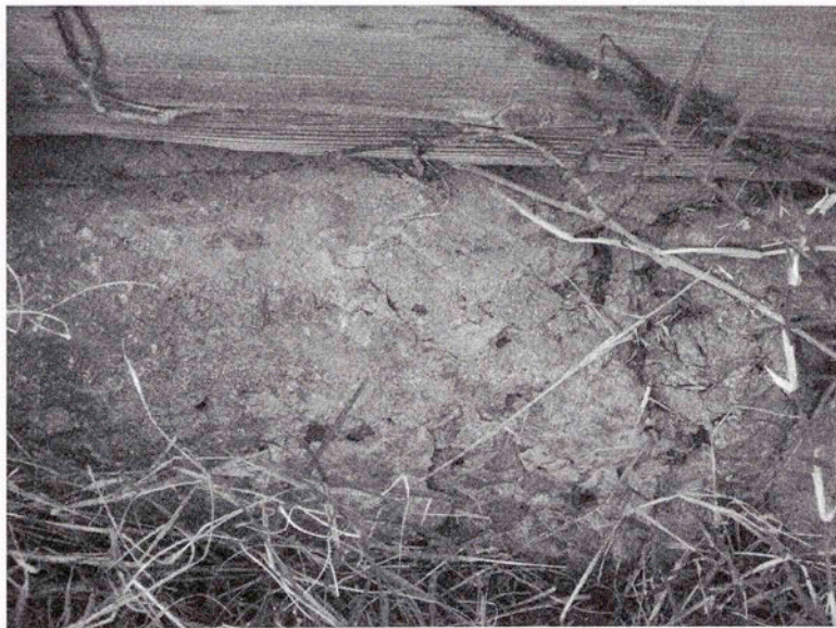
Concrete foundation mixed with red fieldstone.
