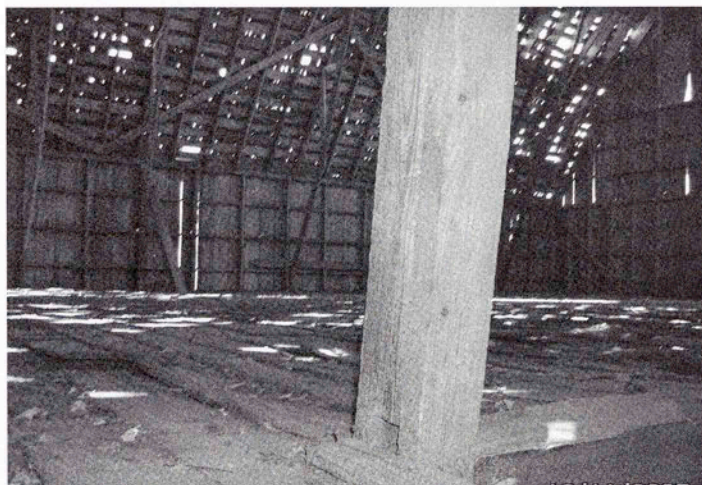
Fig. 5.57 Hayloft floor in the Claus Rohwer barn. (Photo by Lynda Ramsey)
