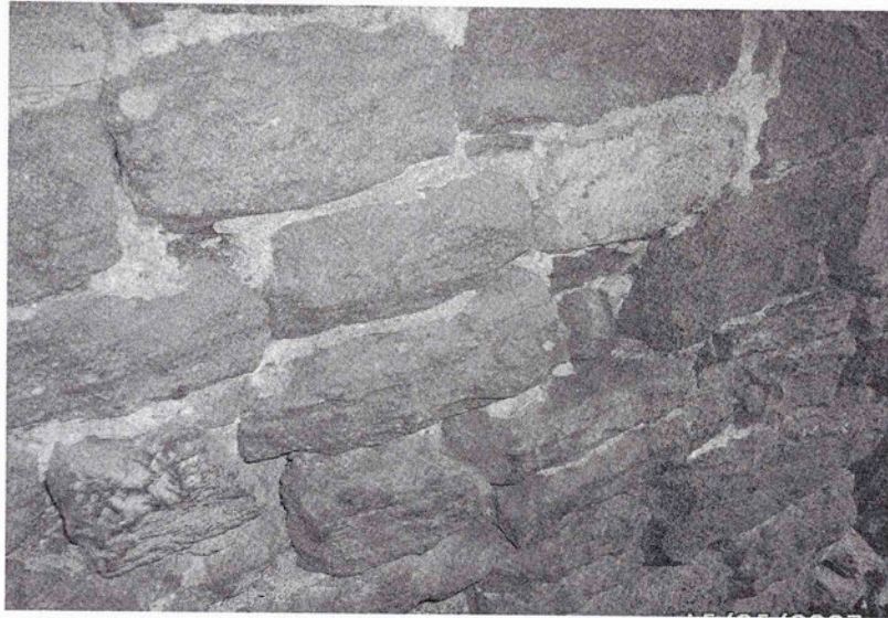
Fig. 5.33 Red sandstone brick wall in Martin Stadler and Tom Beck's barn. (Photo by Lynda Ramsey)
