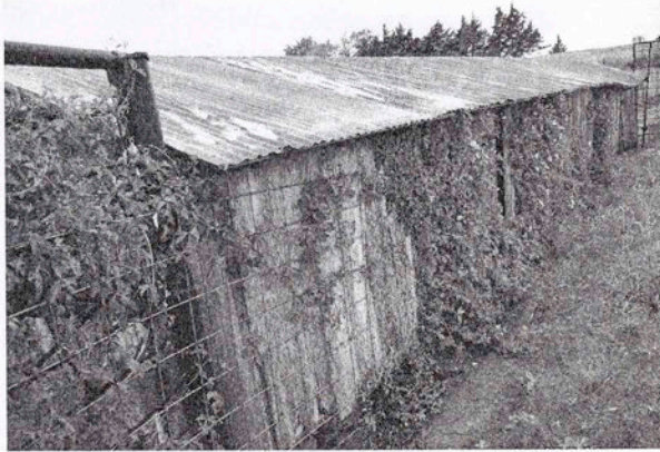
Martin Stadler's Side Hill barn built in 1902. The barn has three hinged doors on the upper slope that open into the hay loft. The barn is built horizontal to the slope and faces the north.
