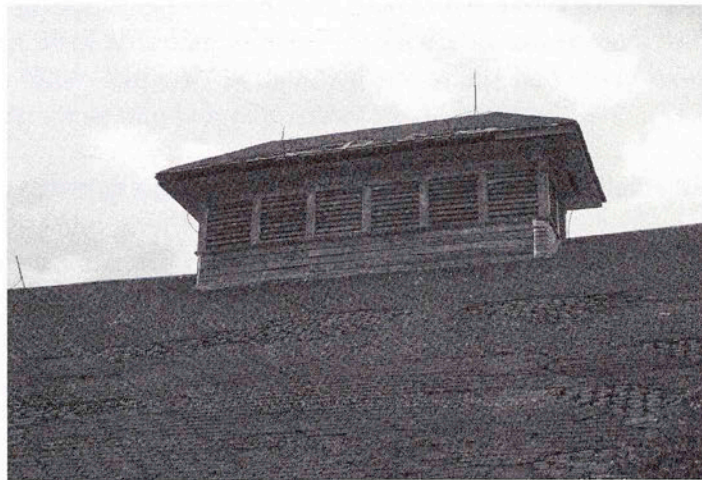
Fig. 5.14 Cupola ventilator on the roof ridge of the Dolezal barn, with Victorian louvers and lightning rods. (Photo by Lynda Ramsey)
