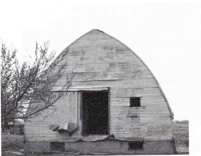
North gothic arch end of F.A. Hall-Mach's bank barn.
