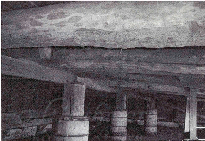
Fig. 5.45 Each post is set into a concrete barrel form sheathed in tin. The tin is fastened around the concrete with iron bands. The heavy axe hewn logs are used as loft floor joists. (Photo by Lynda Ramsey)
