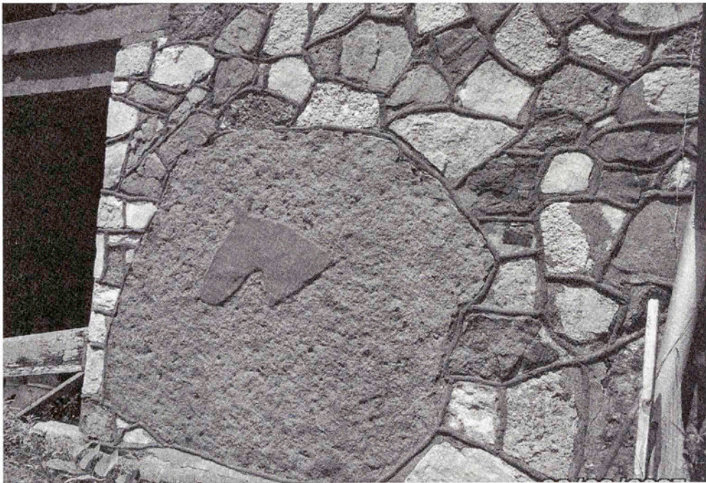
Horse's head placed on stone on both sides of the south entry. Each stone is laid with weeping mortar.
