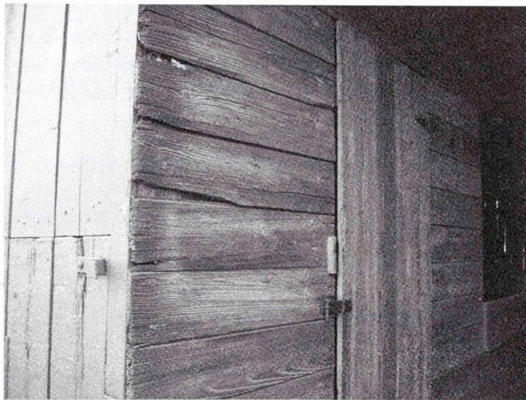
Fig. 5.3 Granary with door and early wooden latch. (Photo by Lynda Ramsey)
