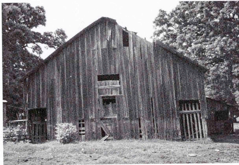
South gable end of the Sober barn.
