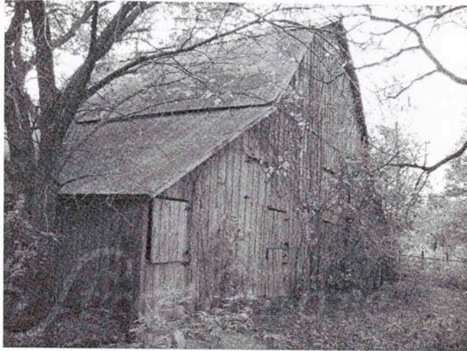
North gambrel end with Dutch doors opening into livestock stalls and walkways. The lengthwise space between the lower gambrel roof and upper gambrel provides ventilation into the loft.
