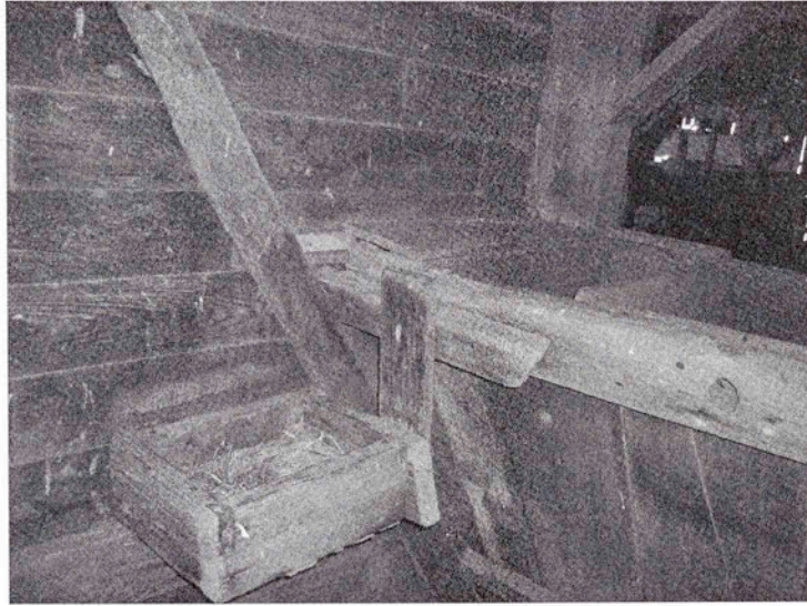
Horse stall in the Charles L. Baker barn provides an area for hay and small wood bins for oats, and salt.
