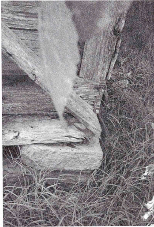
Field stones used as corner support.
