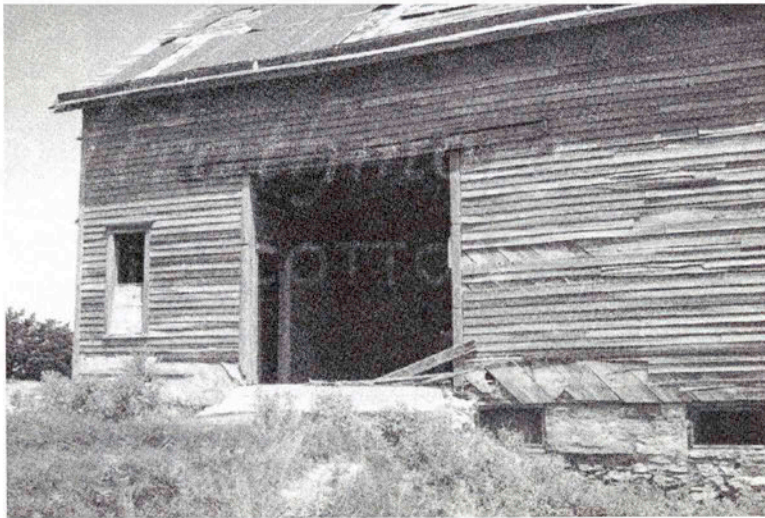
South wagon drive through located on the upper slope.
