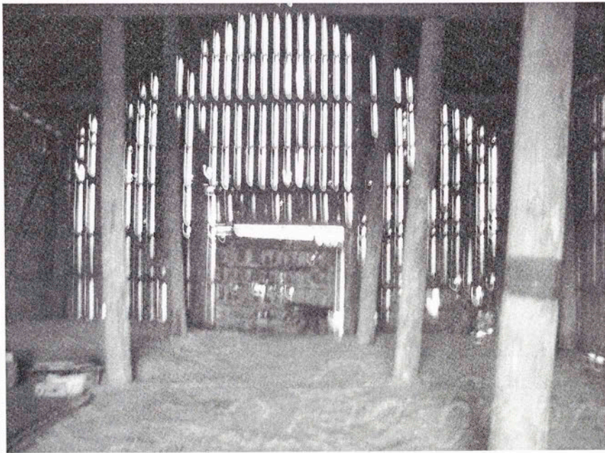
Dirt drive through and hewn support post in Smola barn.
