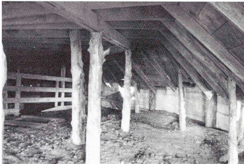
Fig. 5.65 Slanted chutes located around the circumference of the walls allow hay to be dropped into feed troughs from the hay loft. (Photo by Lynda Ramsey)
