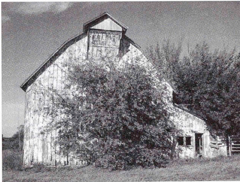
East gable end of the Bollenbach's barn.
