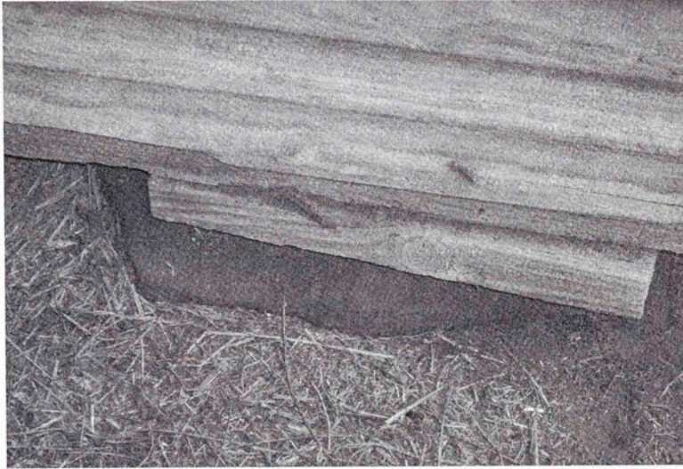
Red fieldstone used to support the floor of the granary inside the barn.
