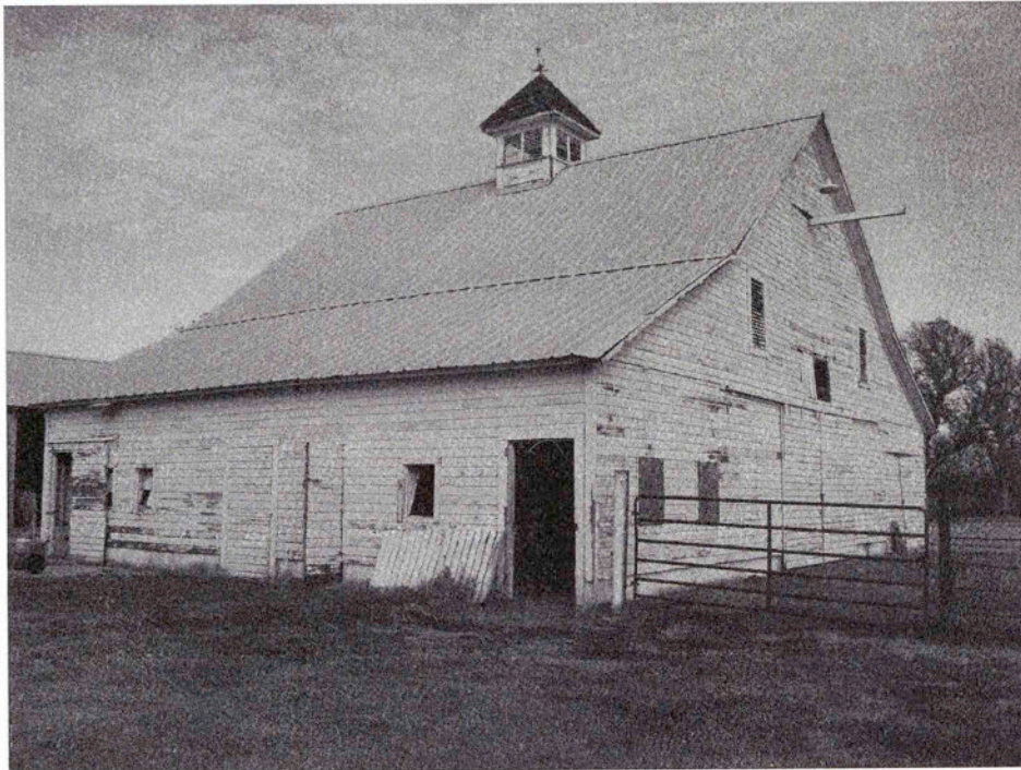
Southwest side of Vaught and Groce barn. Hayfork extension on south gable, and Victorian cupola with a wind vane.
