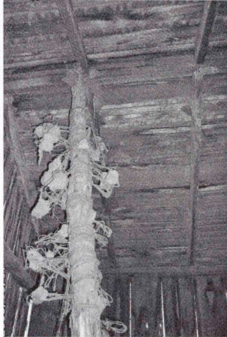
Fig. 5.38 A bois d'arc post used to give the ridge support in Tom and Edna Beck/Stadler barn. Mud dobbers have made their homes amongst the bailing wire that was twisted around the "Osage orange" post.
