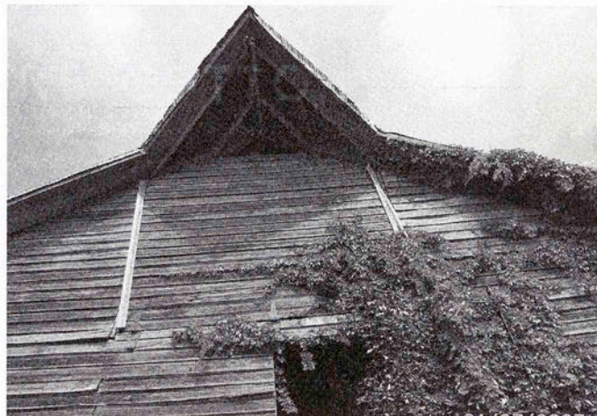
Fig. 5.9 The triangular hay hood on Jack Cooksey's barn, with an attached metal hay track and pulley above the loft door. (Photo by Lynda Ramsey)
