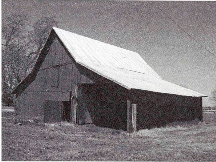
South gable end and east side of Ernie Berousek's barn.
