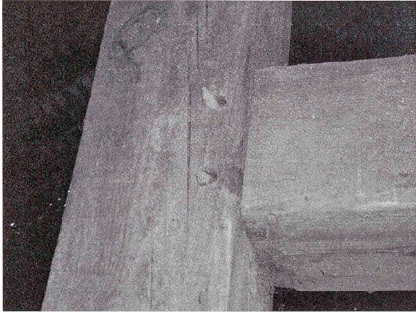
The sharp ends of the peg or treenails through the mortise and tenon joint.
