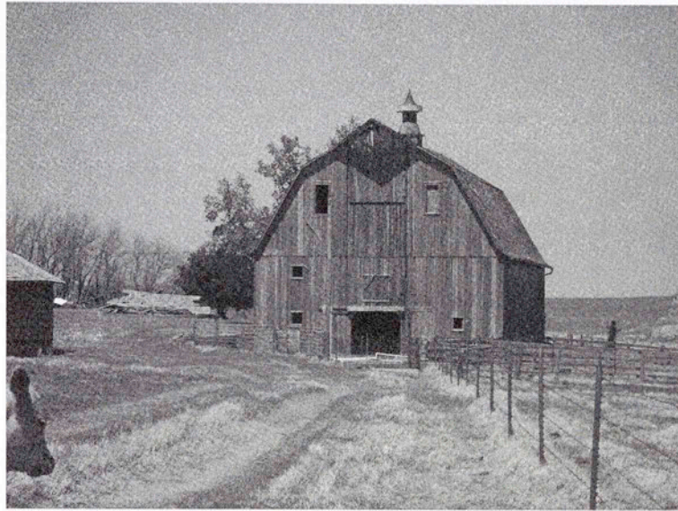
Fig. 5. 54 The Claus Rohwer barn was built 1916 in Altona. The barn has a Dutch gambrel roof, triangular hay hood, and metal ventilator.
