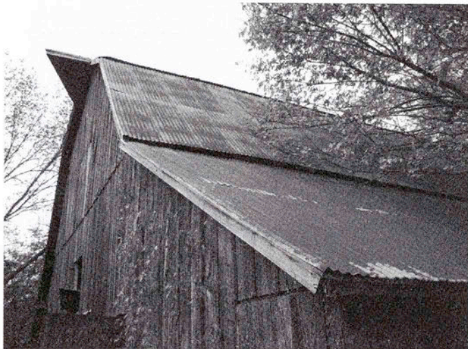
Southeast view of triangular hay hood and ventilation break in the gambrel roof.
