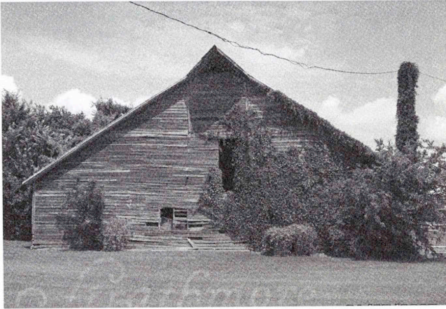
West gable end of Jack and Margarite Cooksey's barn.
