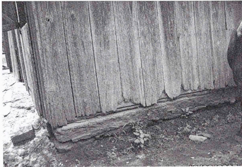
Figure 5.73 Concrete foundation on Elemnhorst and Blaha's barn.
