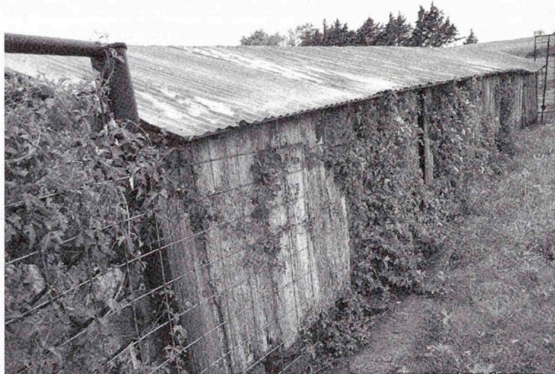
Figure 5.32 The upper level of Martin Stadler and Tom Beck's barn facing the north. There are three doors that open into the loft. The red shale stone is used as the foundation for the wooden upper loft. (Photo by Lynda Ramsey)
