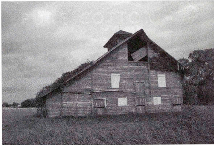
South gable end of Dolezal barn.
