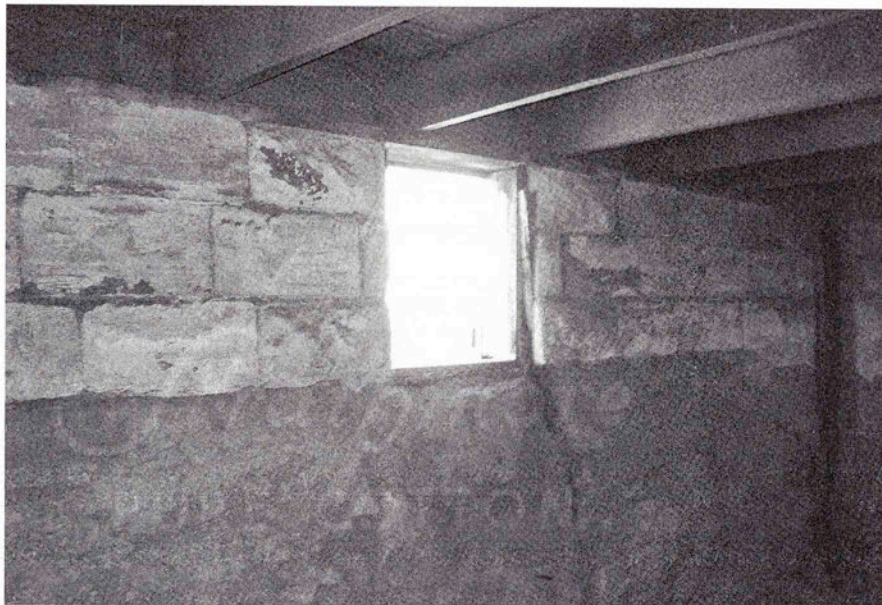
Fig. 5.52 The lower wall is red brick covered with a veneer of concrete plaster. The upper wall level is hollow concrete blocks with a decorative, carved face placed towards the outside. Whitewash has been used to coat the inside wall of blocks. Above, the block masonry wall the floor beams are seated on the wood plate. (Photo by Lynda Ramsey)
