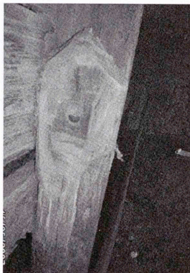
Figure 5.40 A post hewn by a broad axe in the Stadler and Beck barn. (Photo by Lynda Ramsey)
