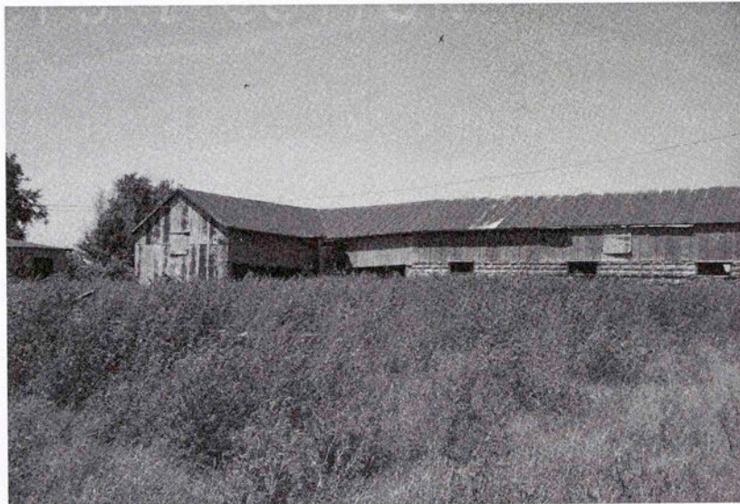
Southwest corner of the Otto Bredel barn.
