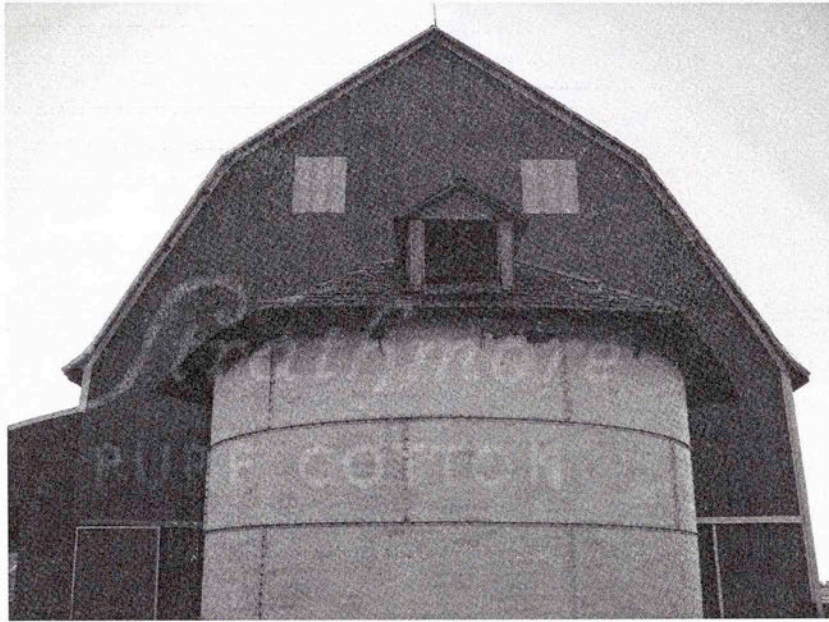
East end of Emmerich's barn where circular metal granary stands with pyramid wood shingle roof and dormer ventilator opening.
