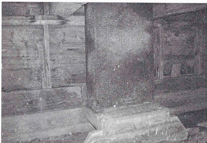
Fig. 5.48 Metal from the discarded ice block containers is used to construct the feed chute that allows grain to travel from the upper loft into the livestock feed troughs. (Photo by Lynda Ramsey)
