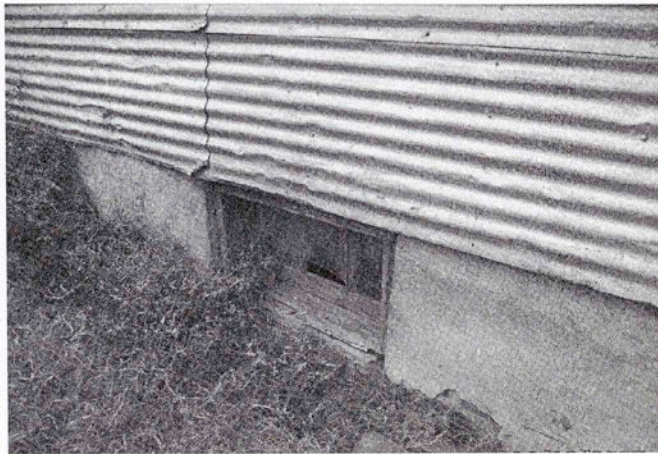
Three pane awning window located in the lower foundation or basement.
