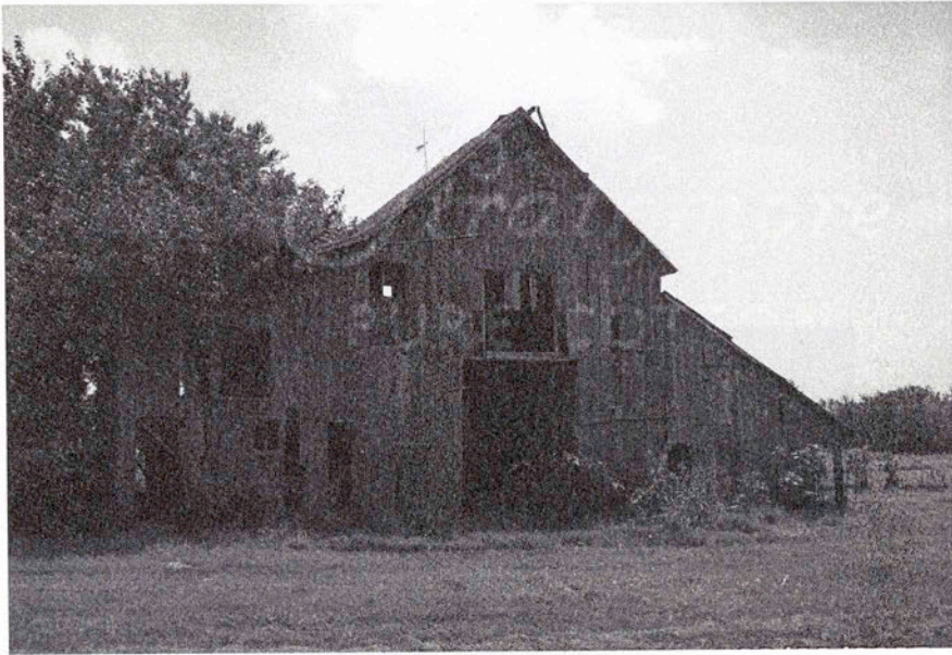
West front of barn.
