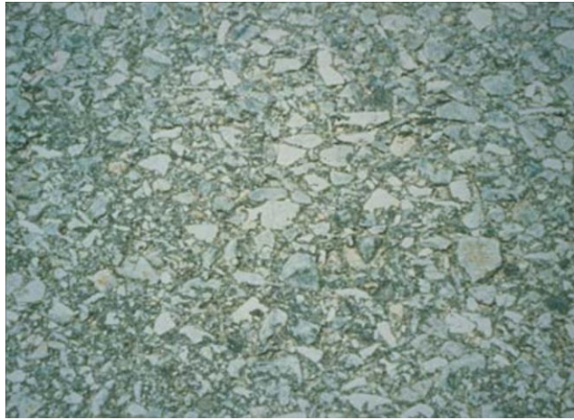
Figure 2.1. Pavement Distress Example – Polished Aggregate
