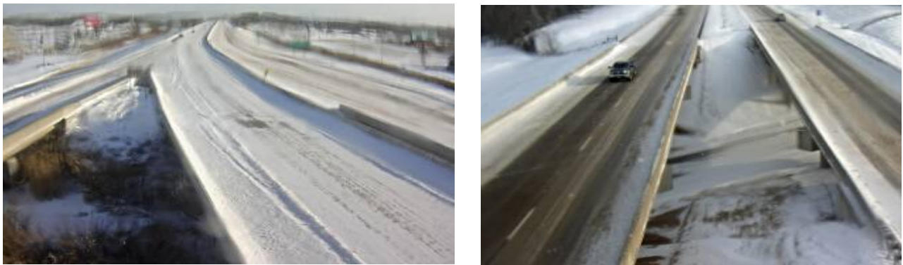
Figure 4-32. Road view difference between neighboring stations 154 and 165.
