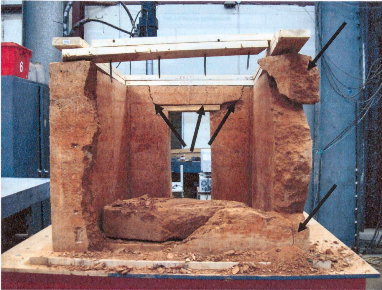
Figure 3.40: Test 3 model after demolition (arrows point to cracks from testing)
