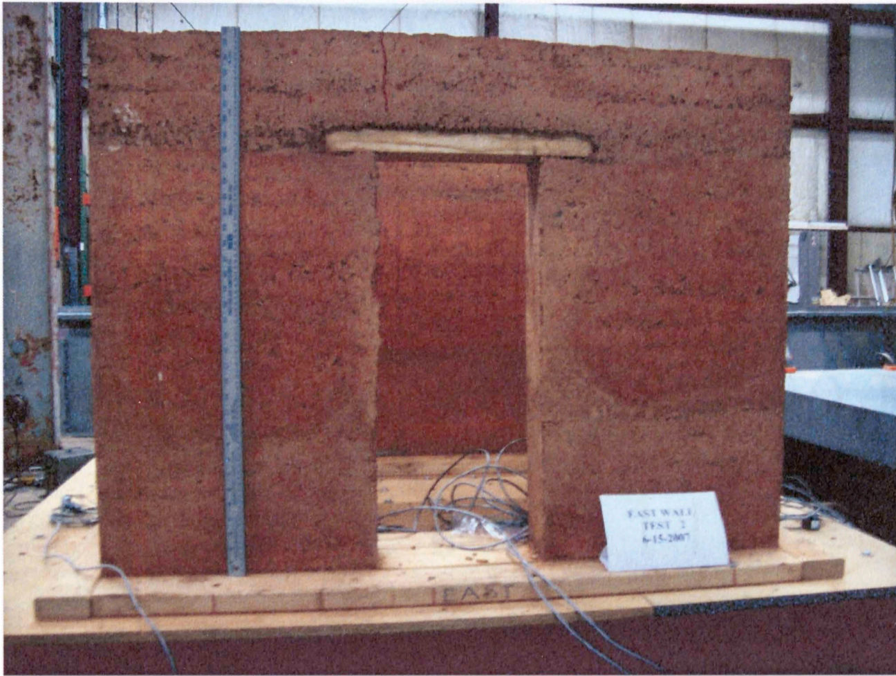
Figure 3.15: Test 2 east wall before test (initial crack above lintel outlined in red) less compacted soil adjacent to edge of lintel
