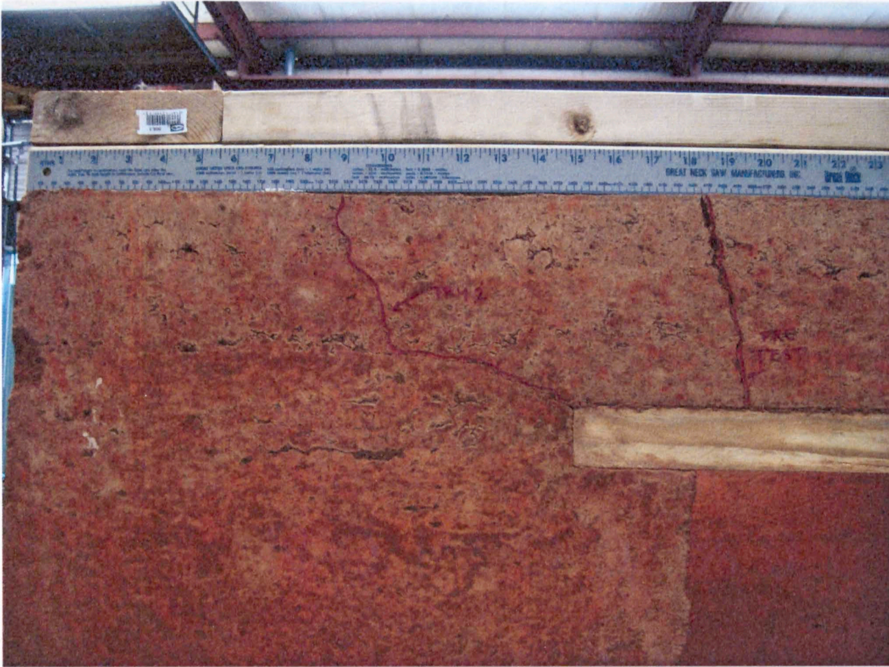
Figure 3.28: Test 3 cracks above lintel near SE corner of east wall
