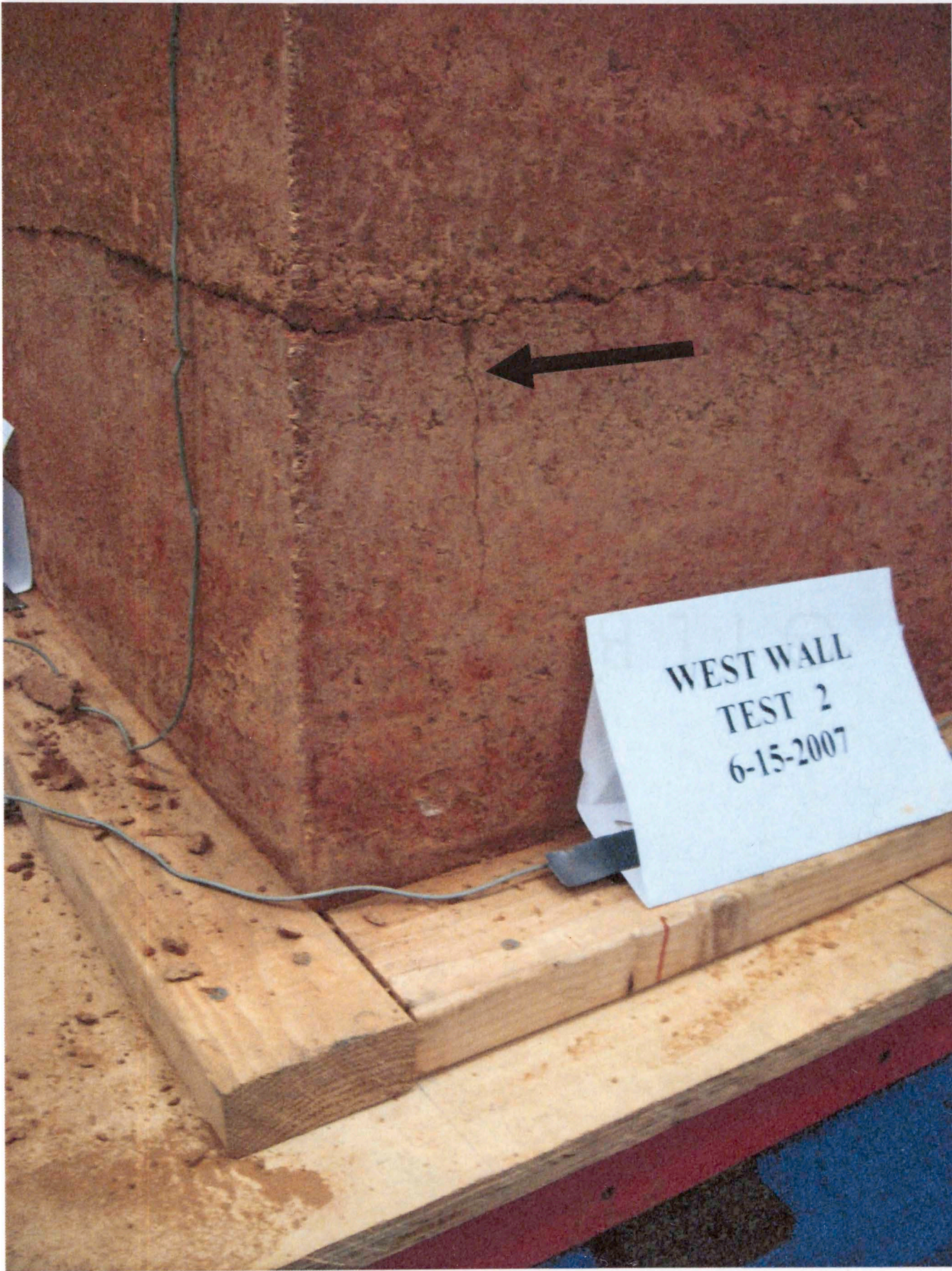
Figure 3.24: Test 2 vertical crack at NW corner below delaminated layer
