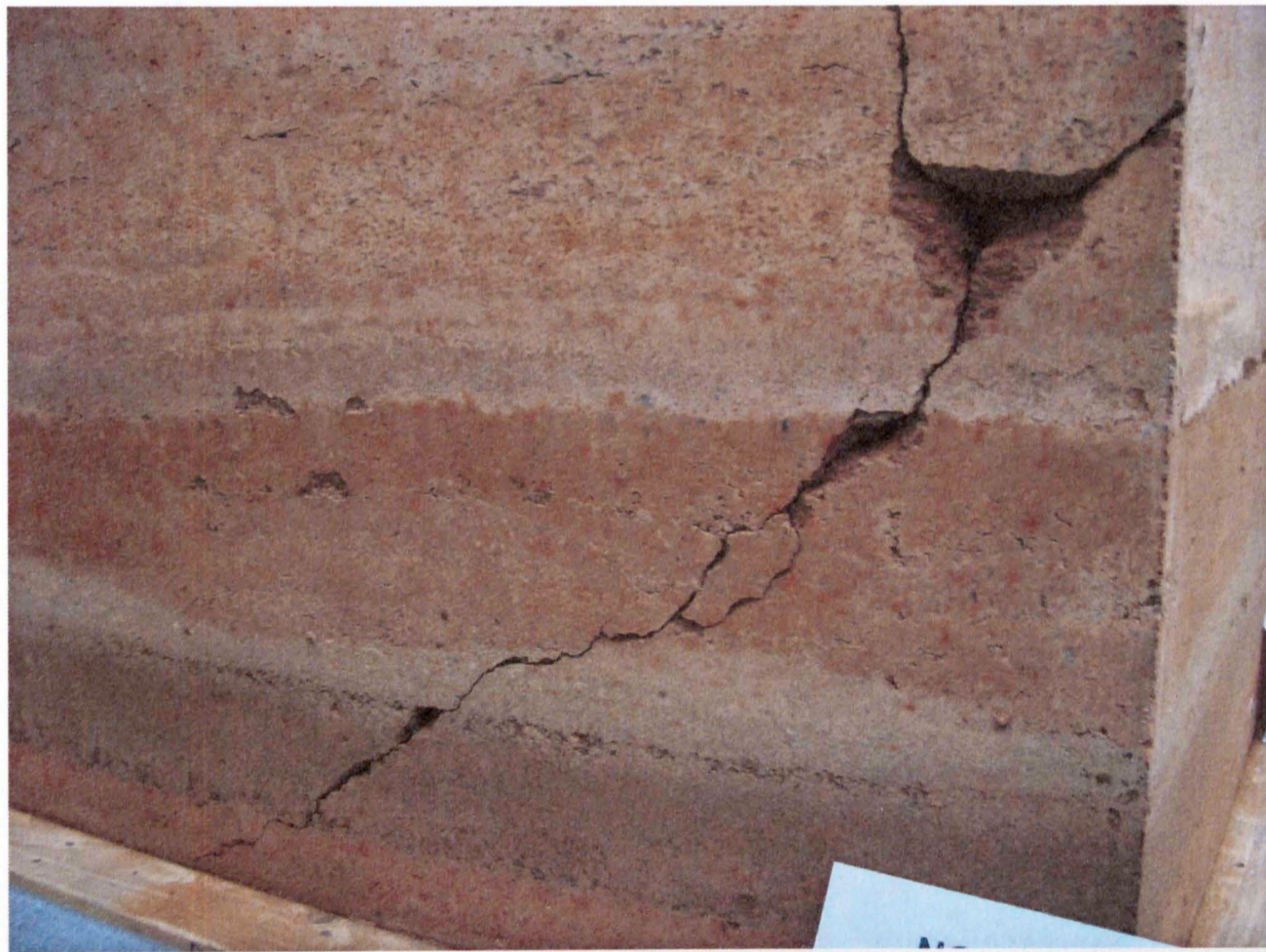
Figure 3.10: Test 1 close up of diagonal crack in lower half of north wall
