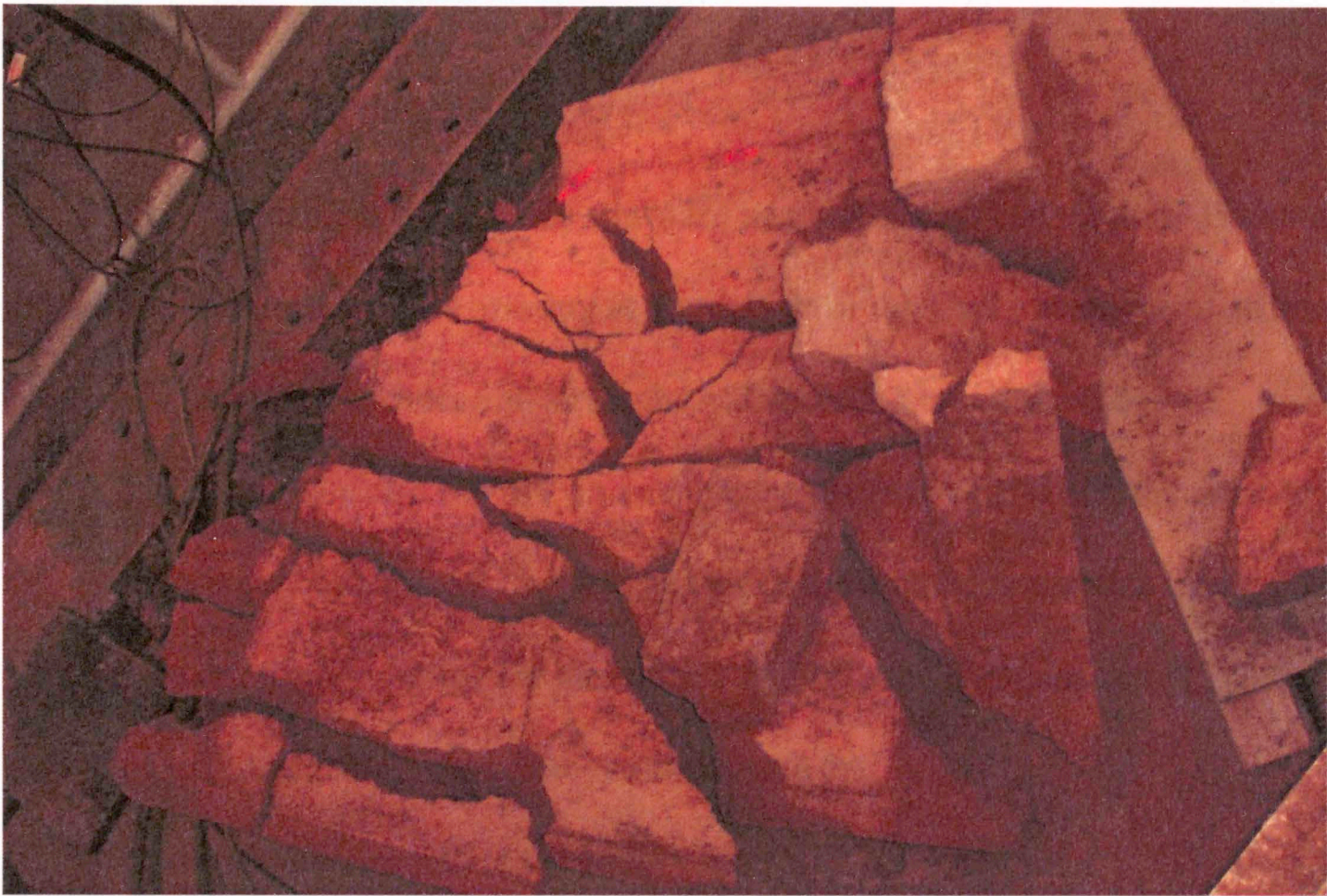
Figure 3.53: Test 4 view of wall that fractured upon impact with the floor
