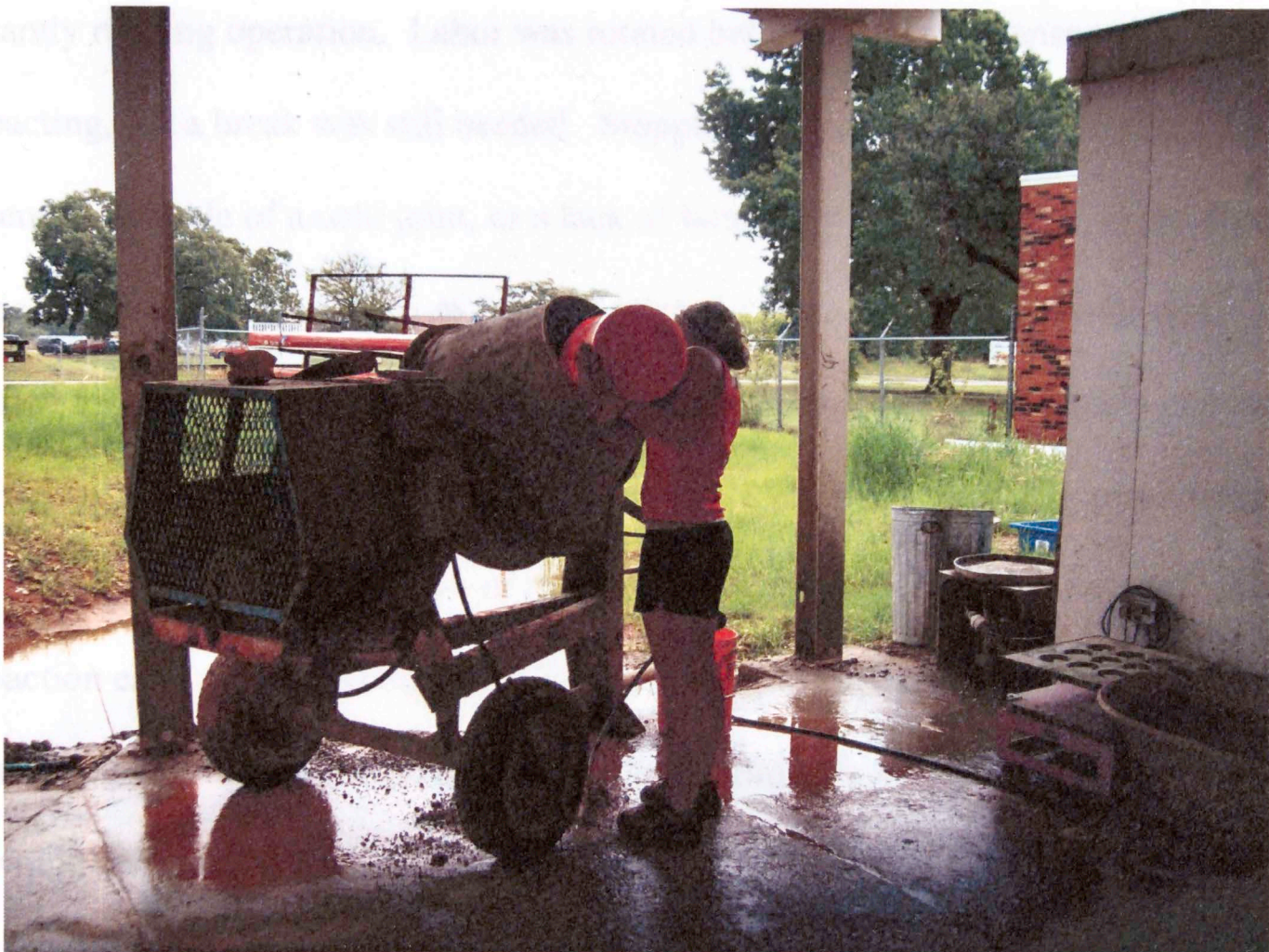
Figure 2.17: Pouring of soil into mixer
