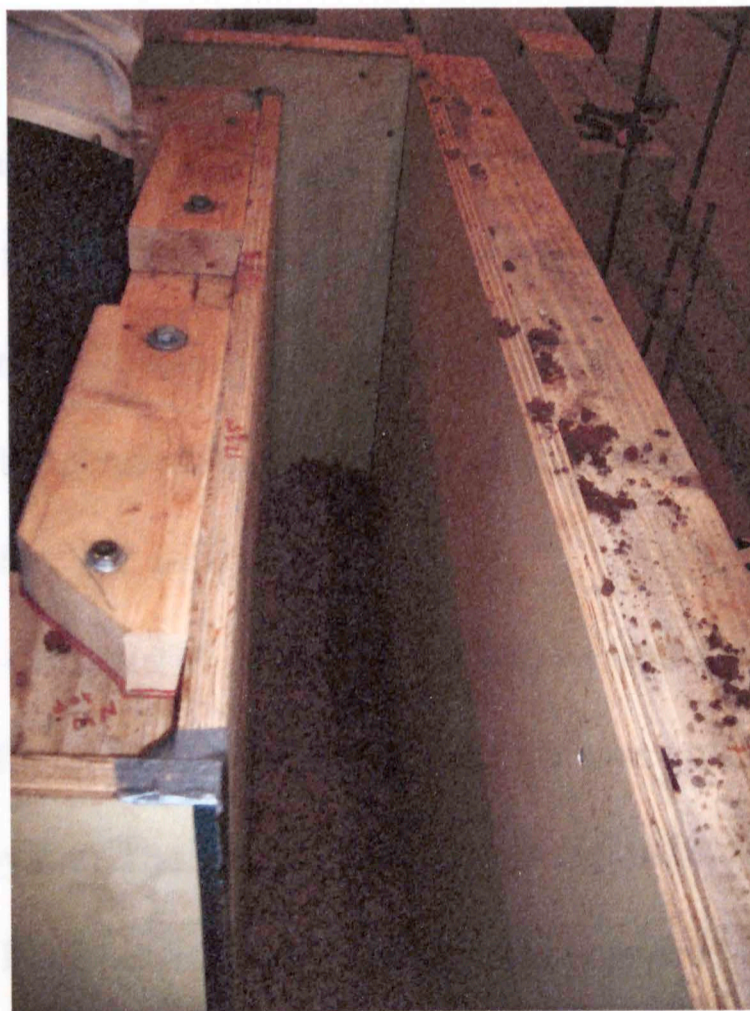
Figure 2.19: View of soil inside formwork prior to compaction
