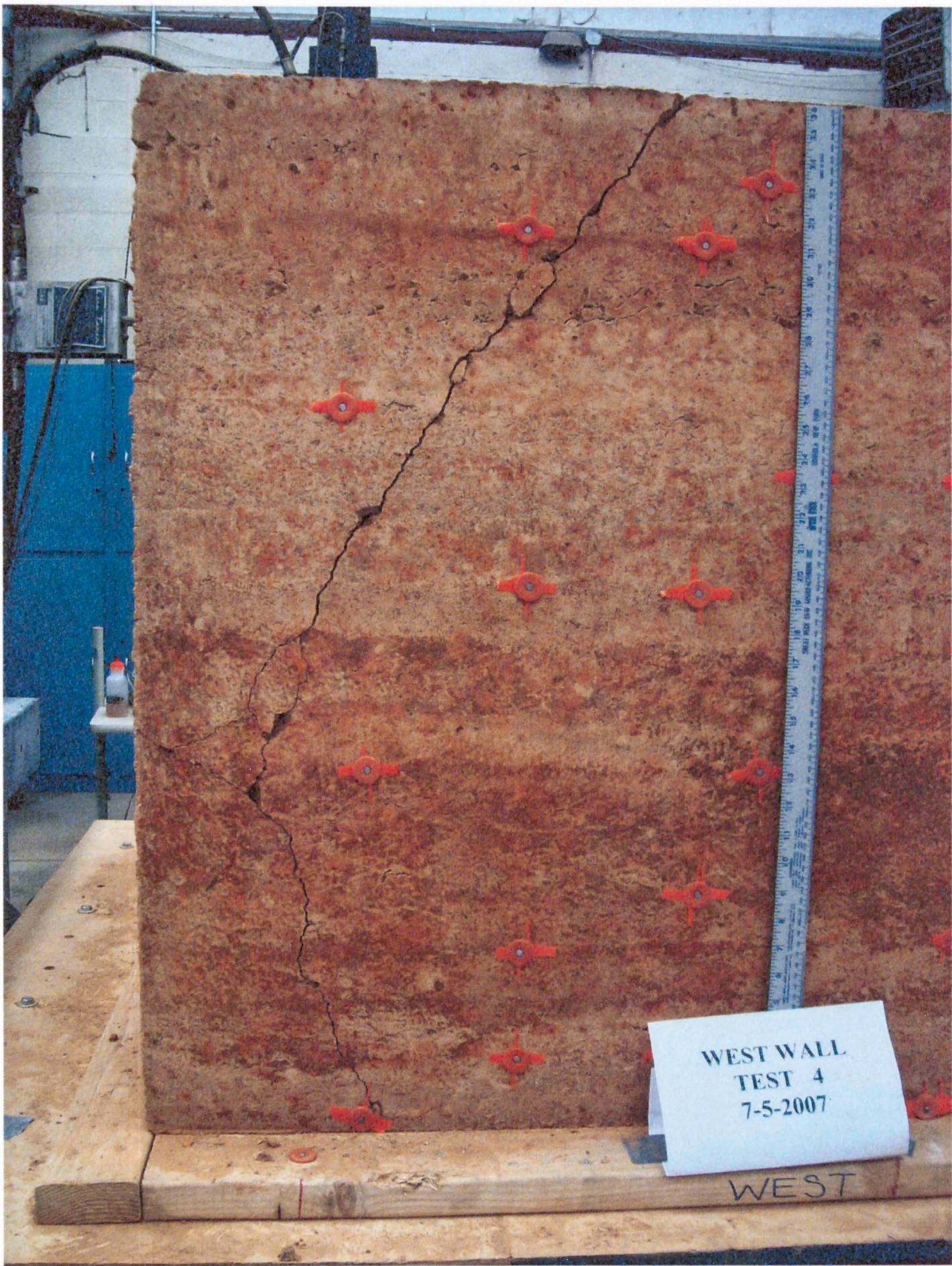
Figure 3.51: Test 4 view of diagonal crack at northwest corner of west wall after test
