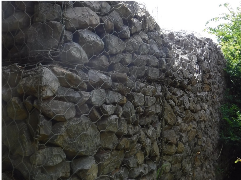
Figure 9: Photo of gabion baskets near Hydro, OK.
