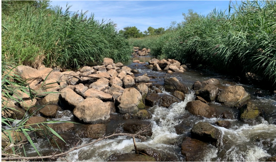
Figure 69: Rock drop structure at site 26
