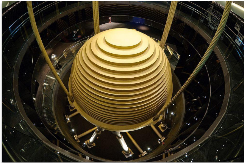
Figure 1.2: Tuned mass damper of Taipei 101 [62].
