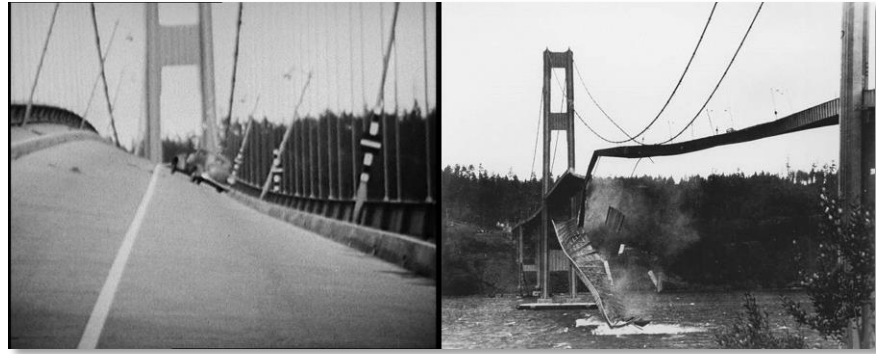
Figure 1.1: Collapse of the Tacoma Narrows Bridge, Washington state, 1940 [64].
