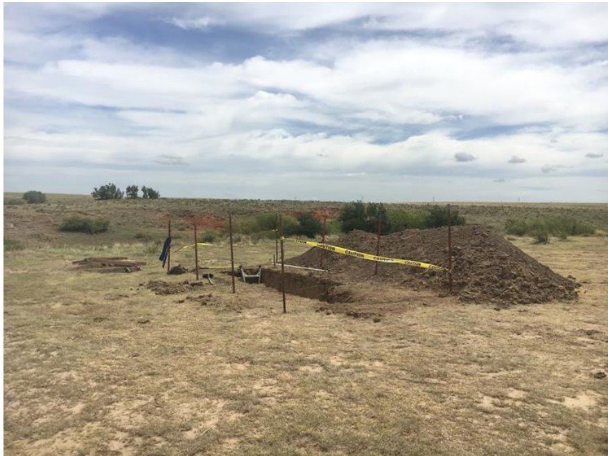
Figure 4-43. Location of backhoe trench, opened and filled in 2018.
