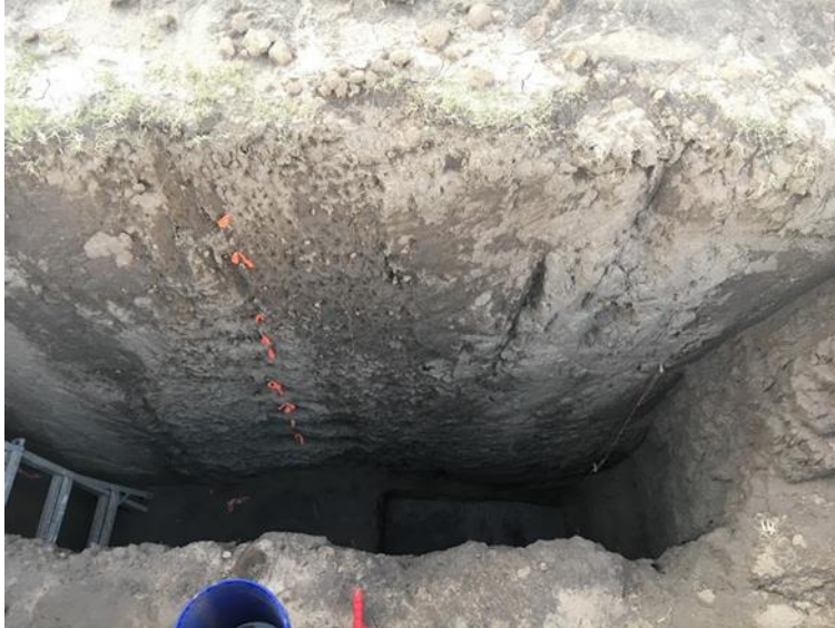
Figure 4-44. Backhoe trench opened and filled in 2018. Shown with tape marking breaks between soil strata.
