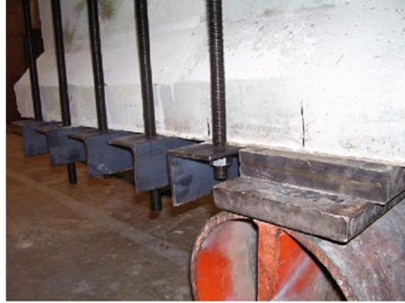
(b) Steel repair and support
