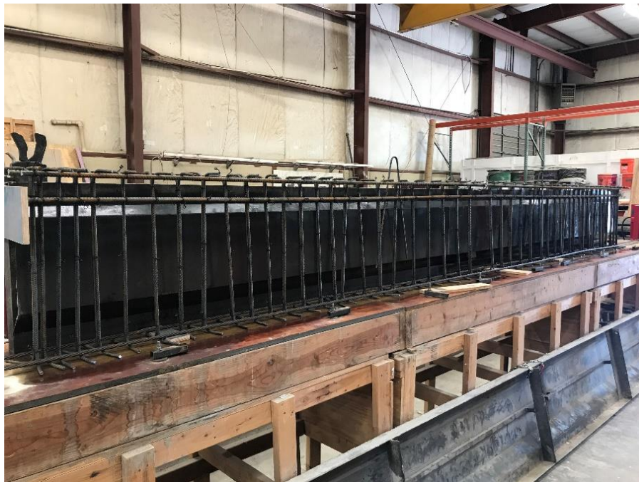
Figure 3.6: Reinforcement cage for a typical girder immediately after prestressing
