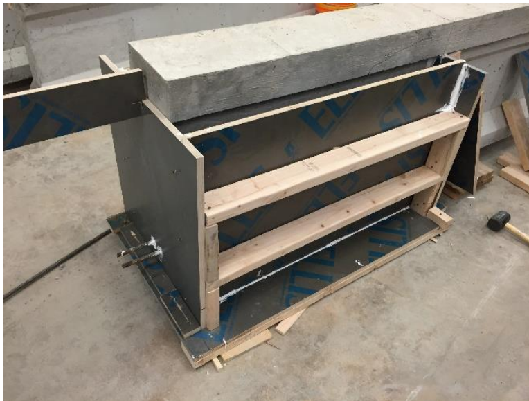
Figure 3.15: Repair formwork
