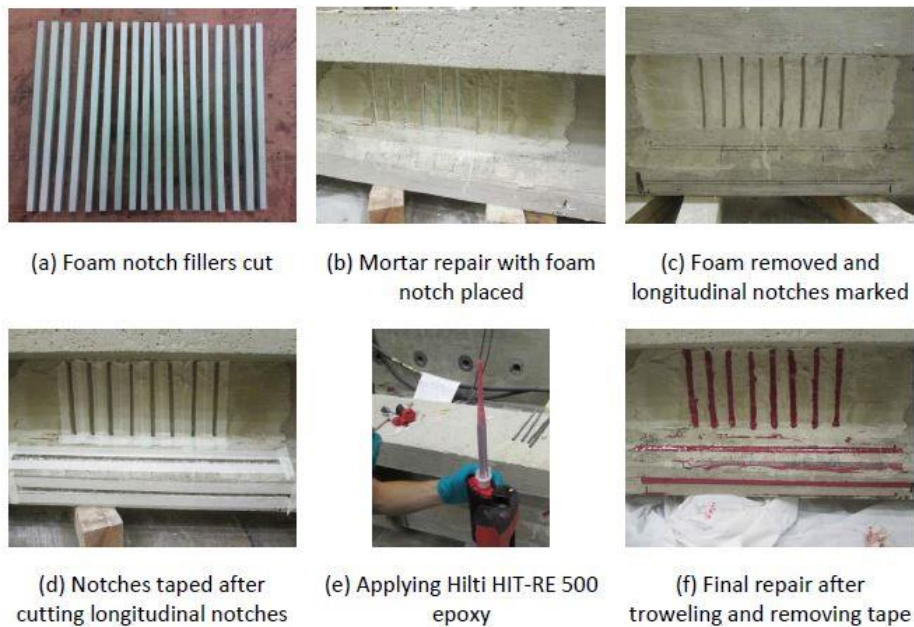
Figure 2.5: Application of NSM bars (Andrawes, 2018)
