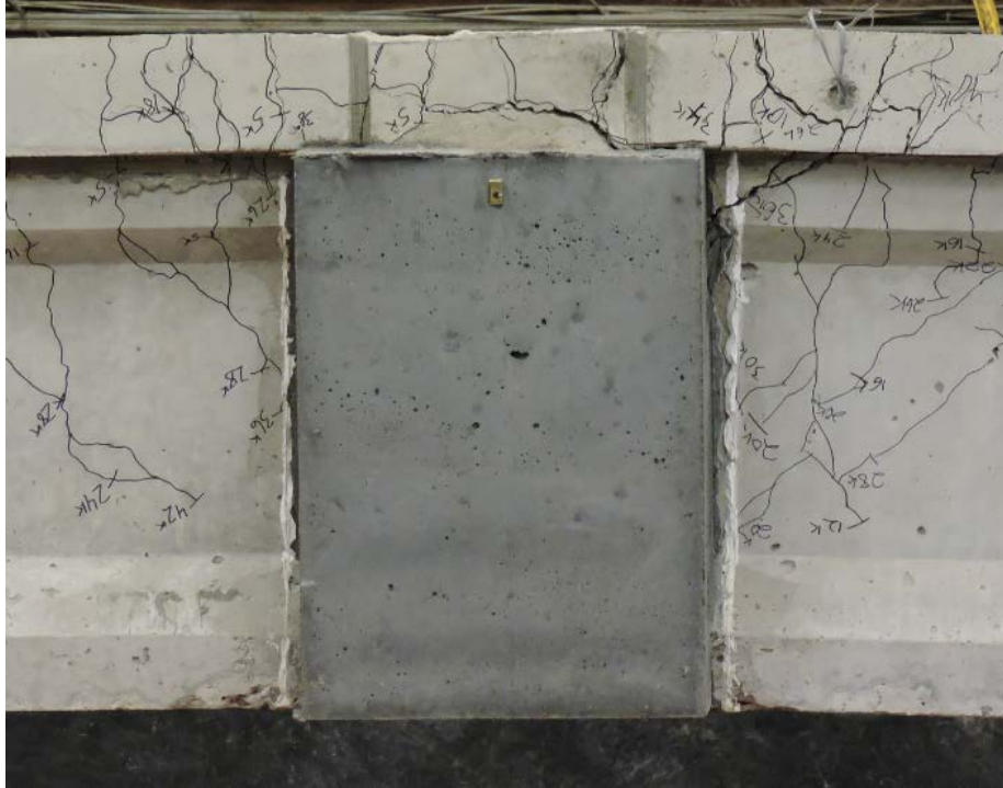
Figure 6-12:R2-J3 Continuity Joint Repair After Testing
