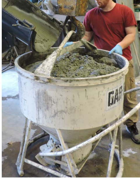
Figure 3-19: Filling Round-Gate Bucket with Concrete
