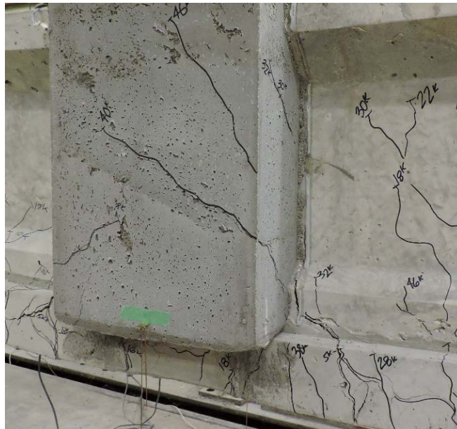
Figure 6-57: R2-PHOS Joint Cracking, Longitudinal and Transverse Faces (Front Right)
