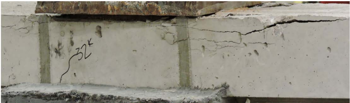
Figure 6-4:R1-J3 Deck Crushing
