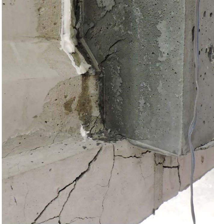
Figure 6-18:R3-J3 Girder-Joint Interface Cracking
