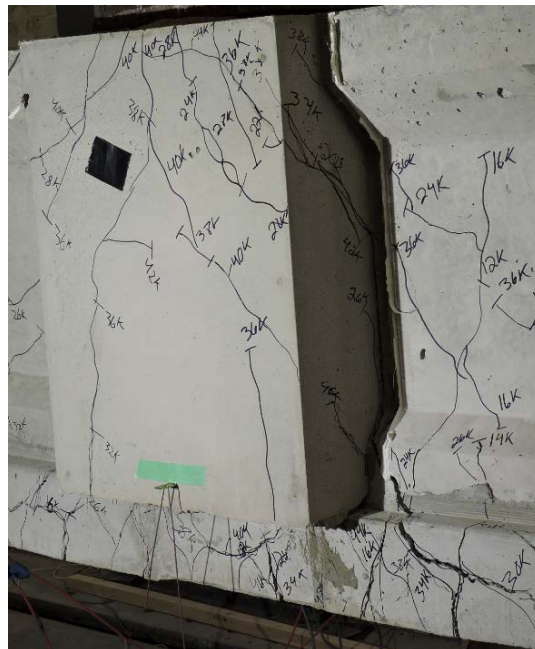
Figure 6-41:R3-FRSCC Joint Cracking, Longitudinal & Transverse Faces (Front Right)
