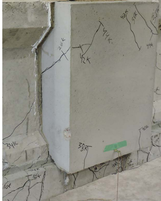
Figure 6-32: R2-FRSCC Joint Cracking, Longitudinal & Transverse Faces (Front Left)
