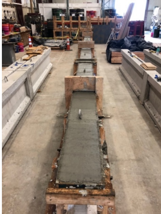
Figure 3-33: Girder-Joint-Girder Specimen After Final Casting
