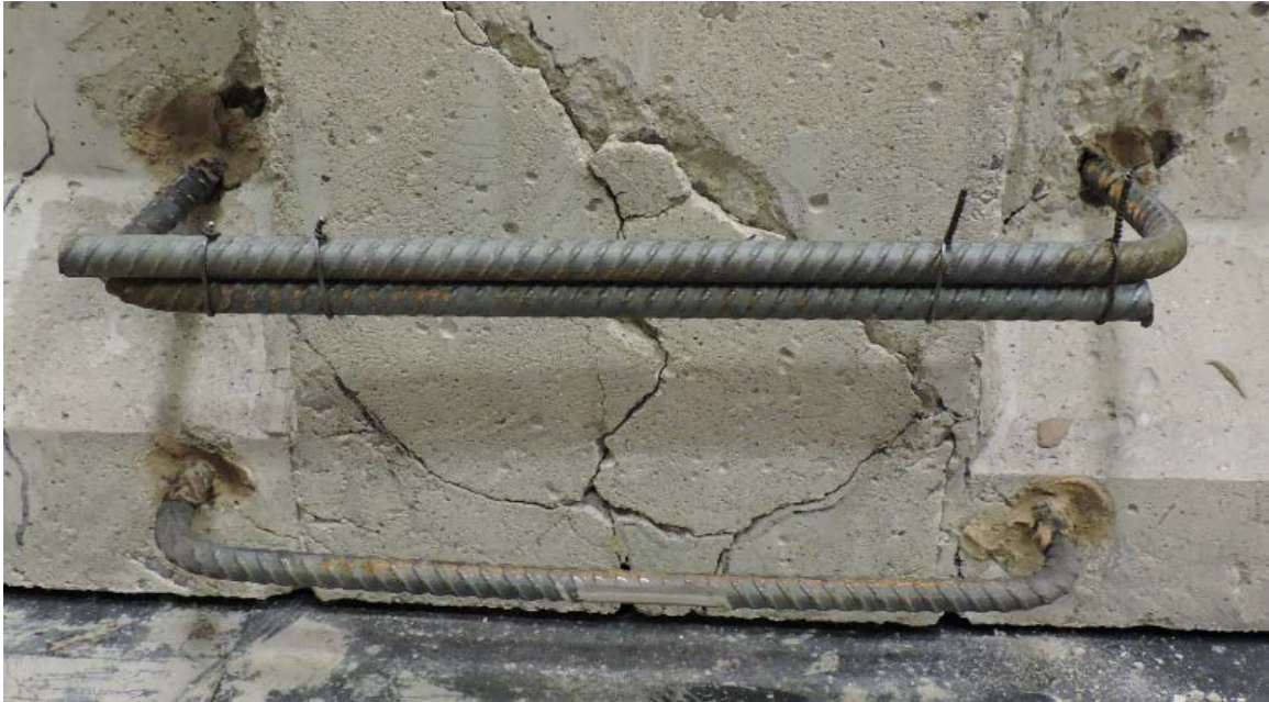
Figure 5-8: Installation of Repair Reinforcement
