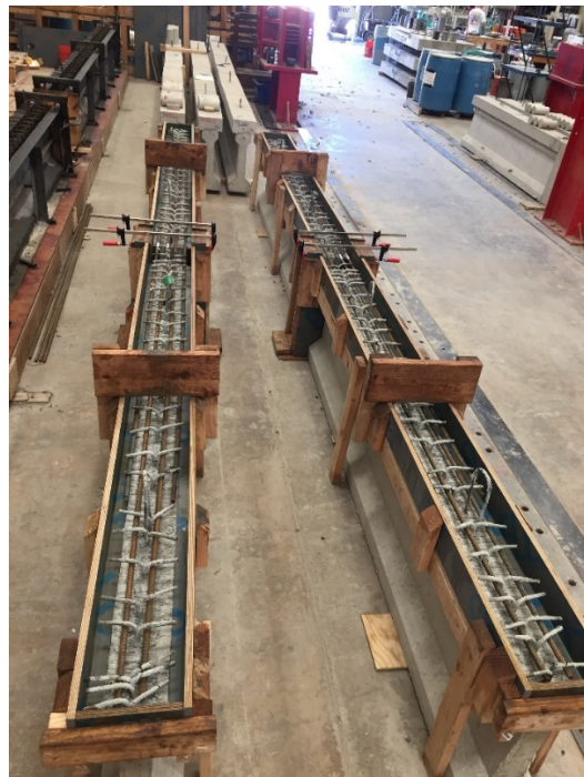
Figure 3-31: Two Girder-Joint-Girder Specimens Prior to Casting
