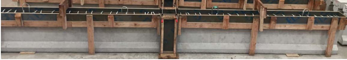
Figure 3-25: Deck Formwork
