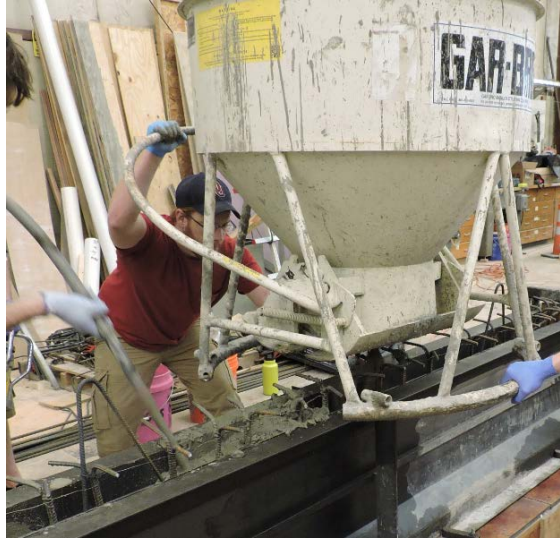
Figure 3-20: Pouring & Vibrating Concrete into Girder Formwork
