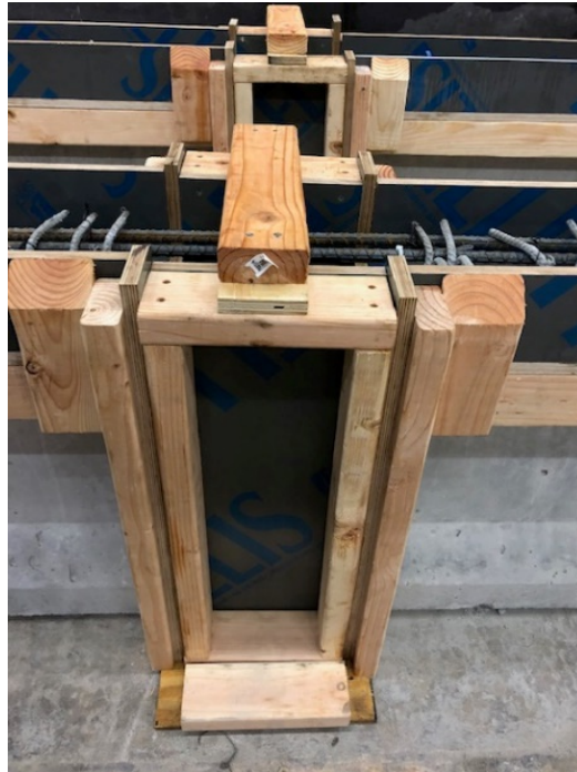
Figure 3-24: Continuity Joint Formwork
