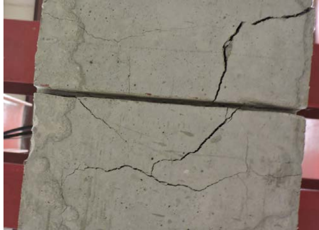
Figure 4-30:R1-J3 Bottom Joint Face Initial Cracking
