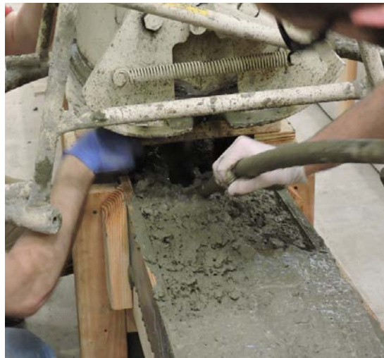
Figure 3-32: Vibrating the Joint During Casting
