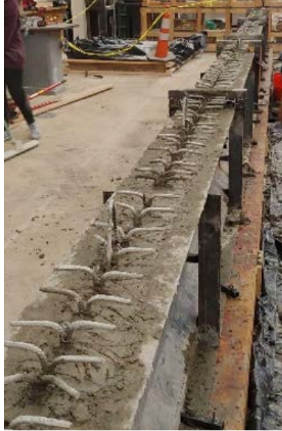
Figure 3-21:Completed Girder Casting
