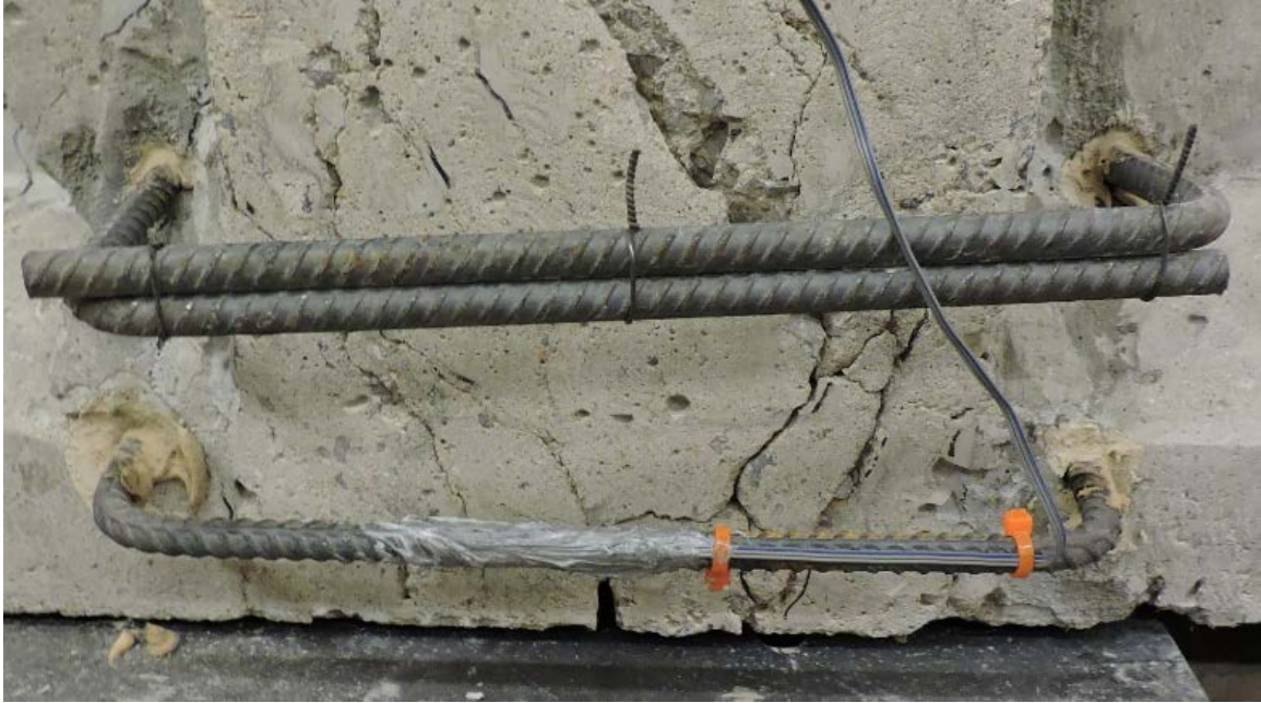
Figure 5-10: Strain Gauge Installed on Repair Reinforcement
