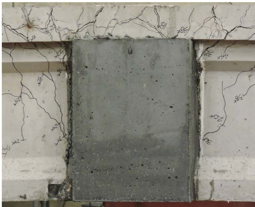
Figure 6-19:R3-J3 Continuity Joint Repair After Testing
