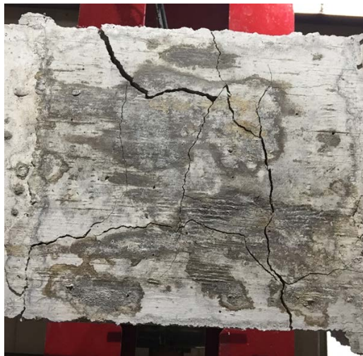
Figure 4-54:R3-PHOS Bottom Joint Face Initial Cracking
