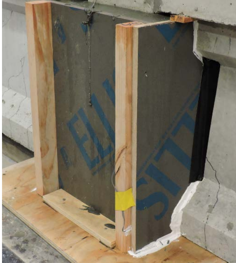
Figure 5-12: Repair Joint Formwork Final Setup
