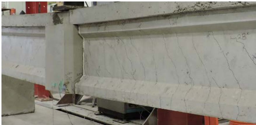
Figure 6-23:R1-FRSCC Shear & Flexural Cracking
