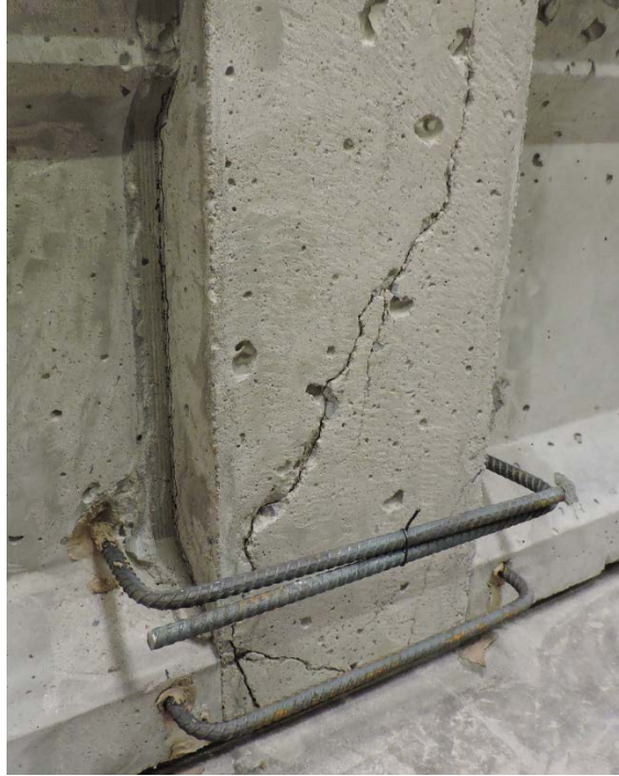
Figure 5-9: Roughened Surface of Areas to Be Repaired
