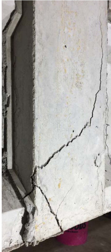
Figure 4-38:R1-FRSCC Front Joint Face Initial Cracking
