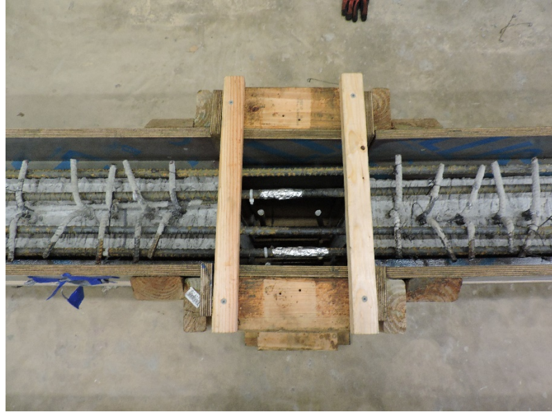
Figure 3-30: Top View of Continuity Joint Prior to Casting
