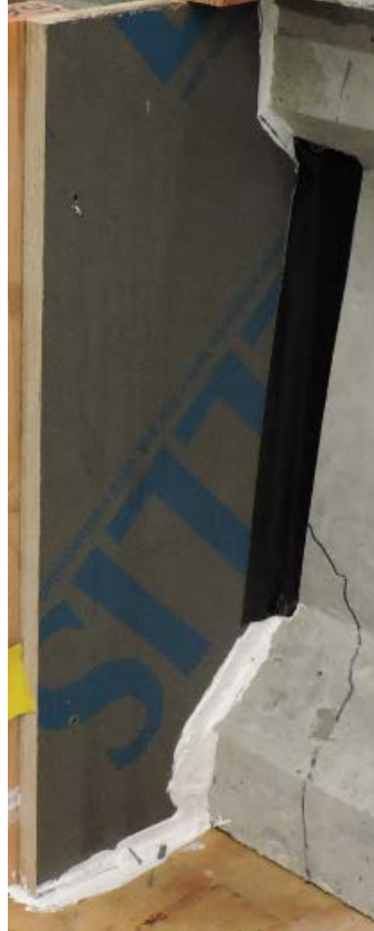
Figure 5-11: Repair Formwork for Side Face
