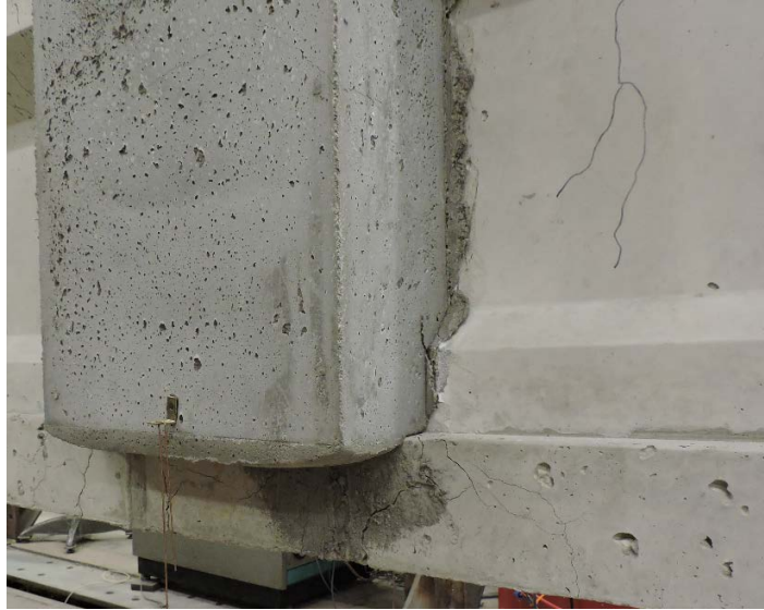
Figure 6-68:R3-PHOS Joint Transverse Face Cracking (Back Right)
