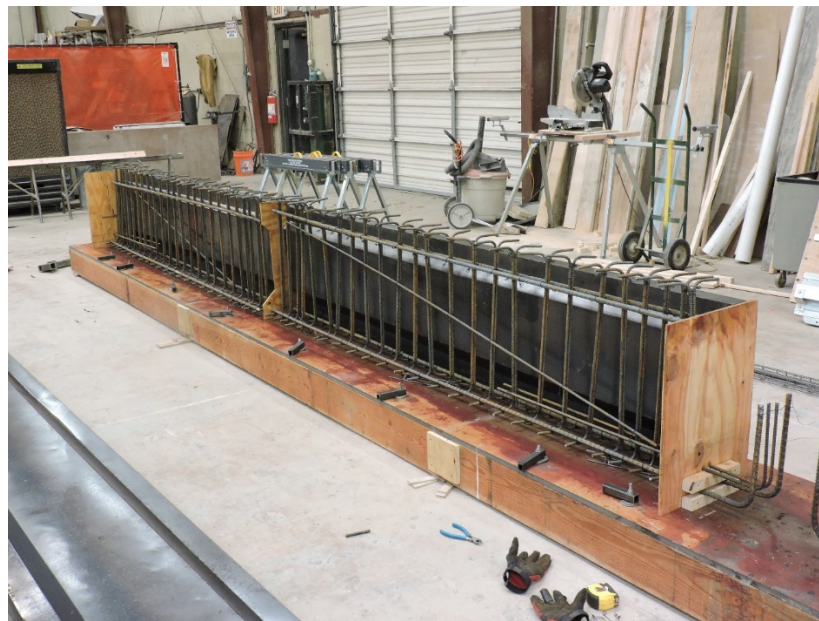
Figure 3-15: Rebar Cages Within Formwork
