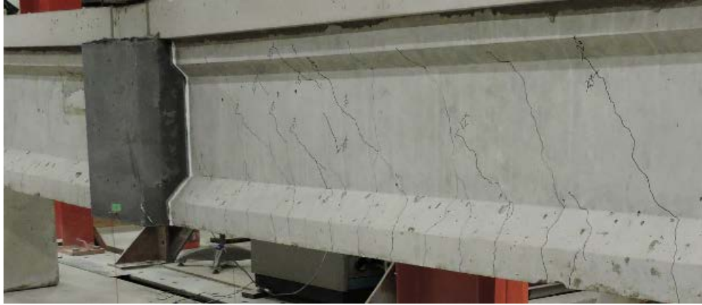
Figure 6-1:R1-J3 Shear & Flexural Cracking
