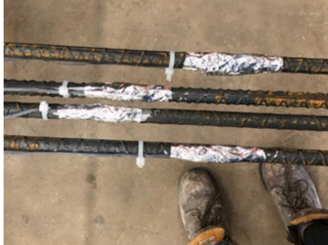
Figure 3-28: Strain Gauges Attached to Longitudinal Reinforcement Ready for Install
