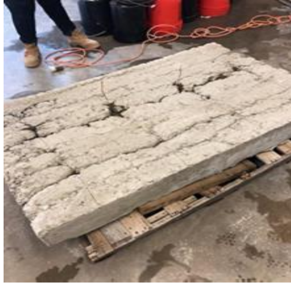
Figure VII.A.I: Back side of Fall 2019 Concrete Wall
