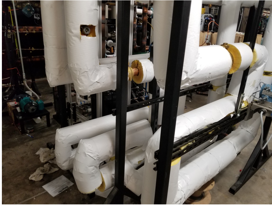
Figure 5.5: Load stand mixing section after modifications
