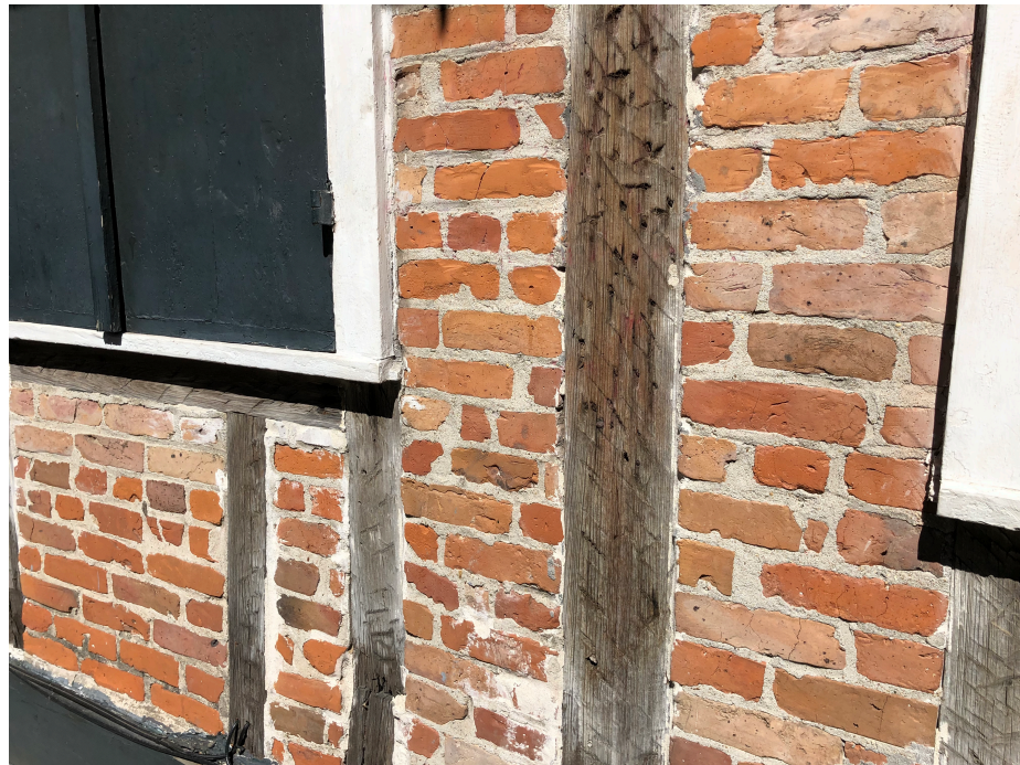
Fig. 9: Examination of the bousillage construction technique on the Creole Cottage
