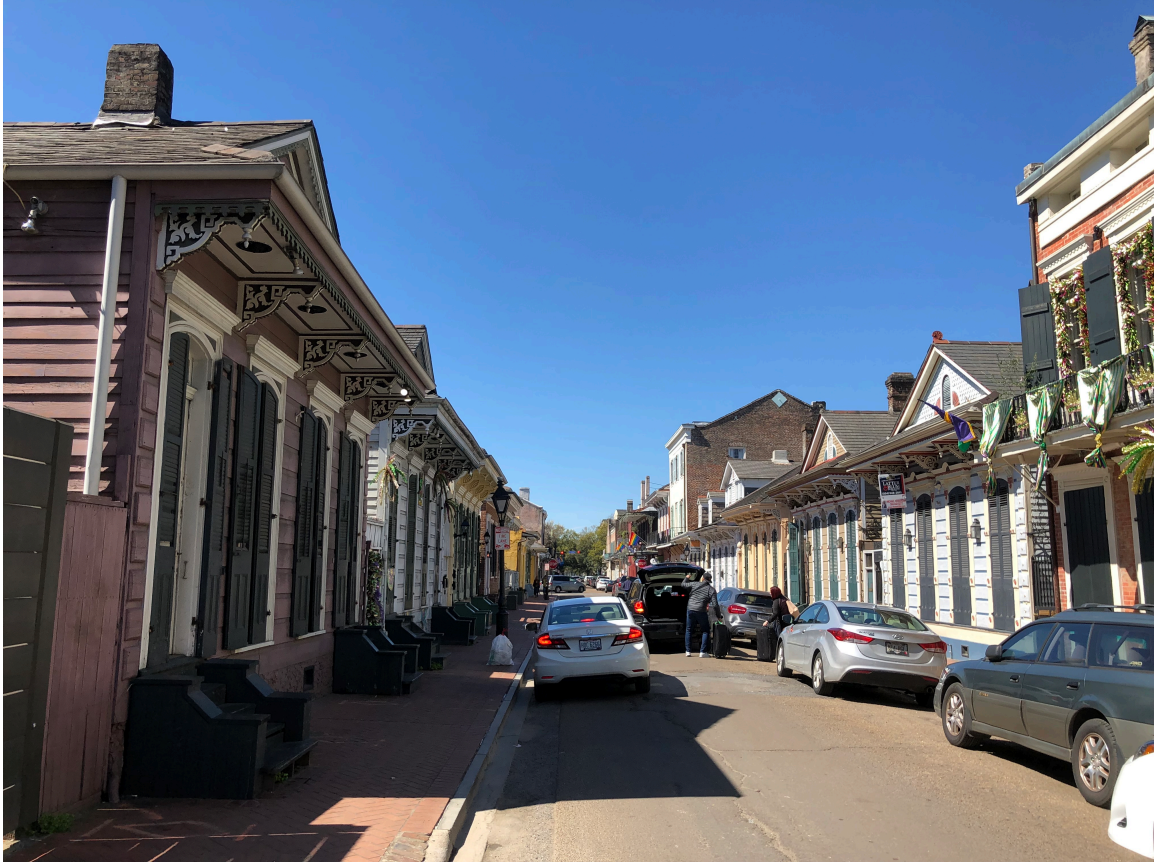
Fig. 18: Tour stop with numerous Victorian Bracket-style Shotgun houses at the intersection of Dauphine St. and St. Peter St. looking toward Rampart St. The Storyville Red Light District.
