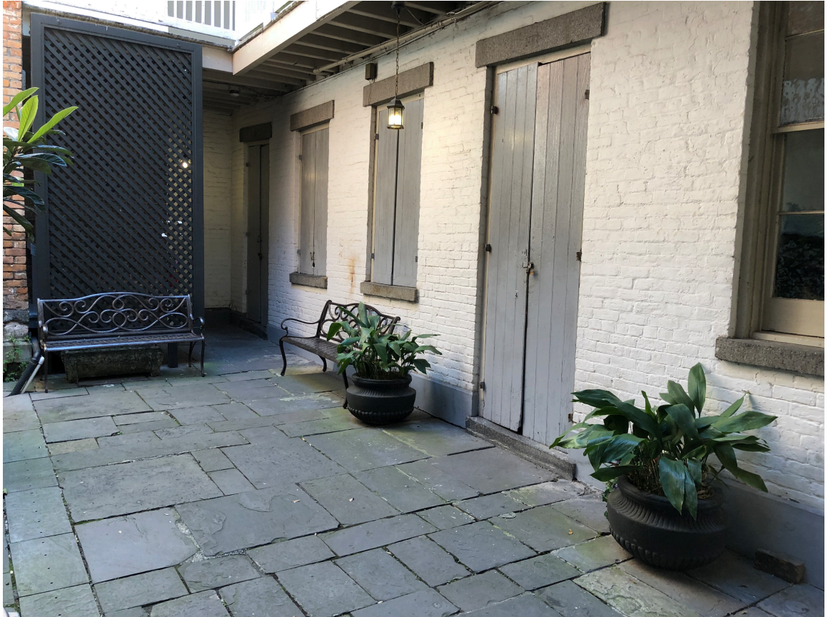
Fig. 3: The courtyard of the 1850 House, where the author begins his tour.
