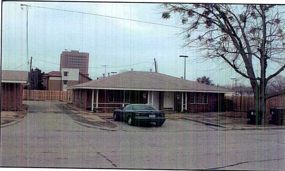
FRONT VIEW OF SUBJECT PROPERTY
