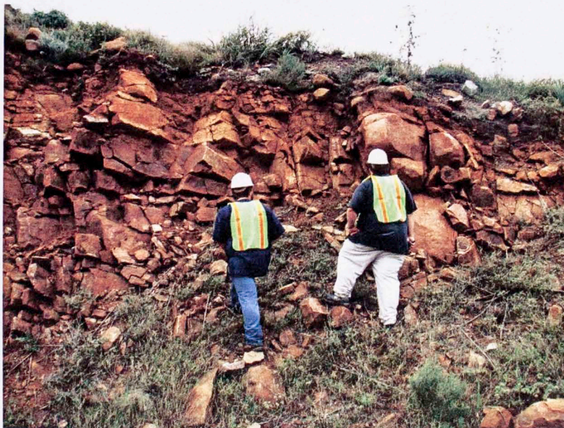
Figure 4.1. Developing tor topography in red granite. Note heavy fracture intensity.
