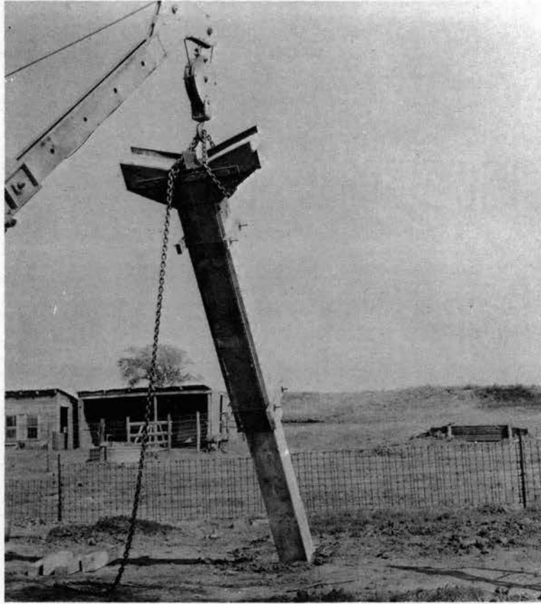
Figure 24. Method of Lifting Precast Column During Erection.
