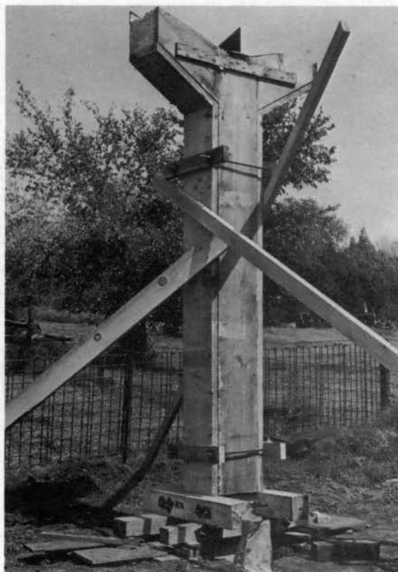
Figure 21. Erected Column Showing Cribbing Clamps.
