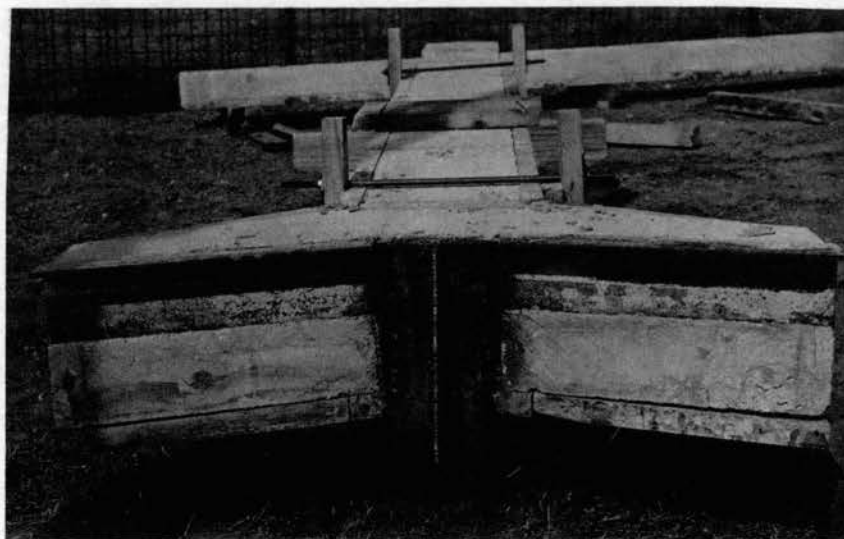
Figure 8. Tie Connection Welded to Bearing Plate on Top of the Column.
