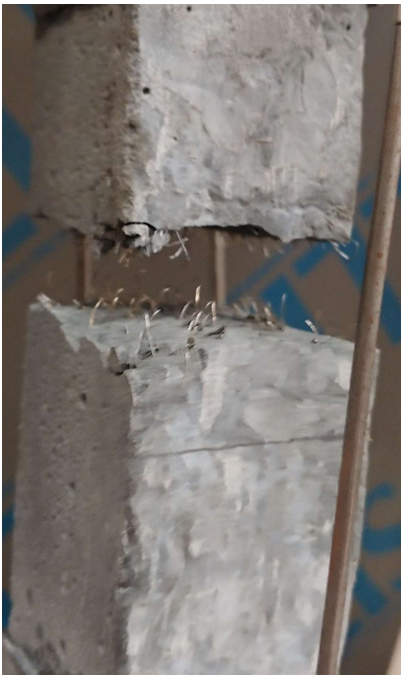
Figure 4.2.2. 6 Crack pattern 1% steel fiber content Specimen 3
